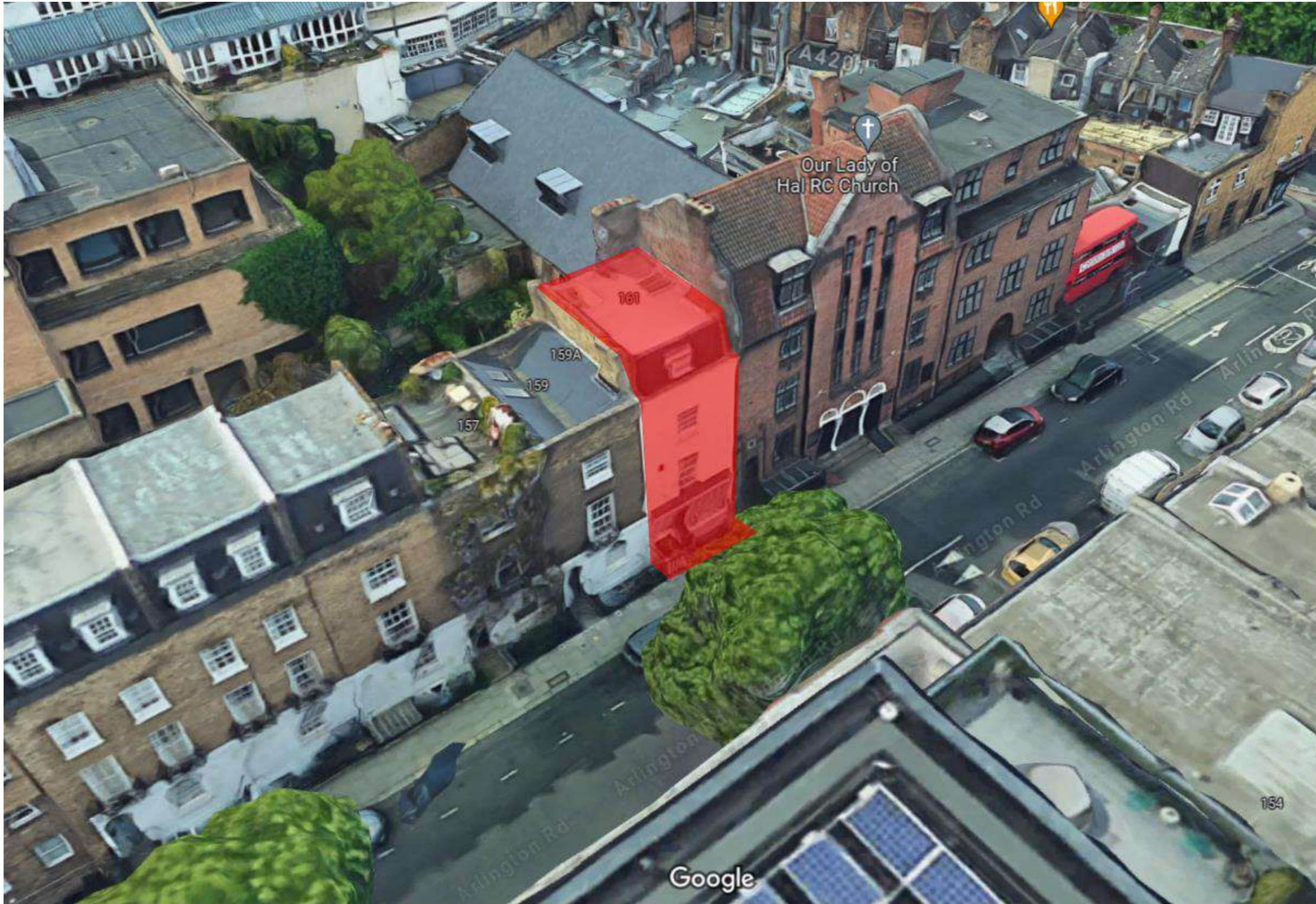
A 4. View of 161 Arlington Road from Front Showing Neighbouring Buildings (Google maps)
