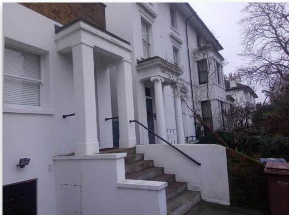
Fig 1.1: Trial Hole 1 Location
