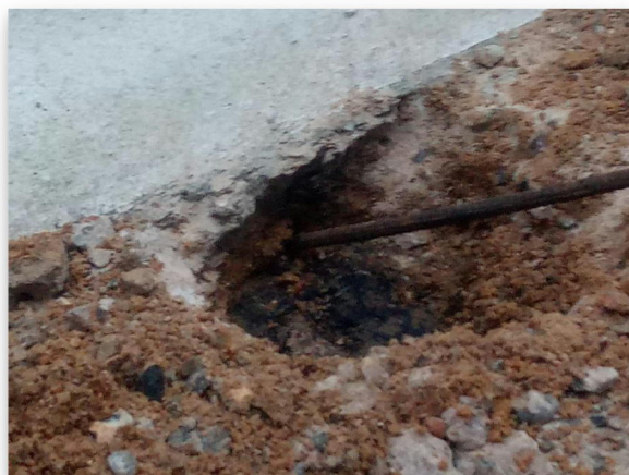
Fig 2.2: Trial Hole 2 Footing
