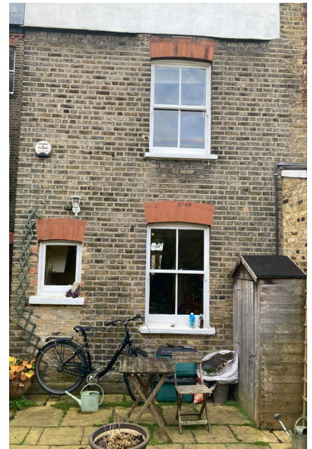
View of rear extension.
