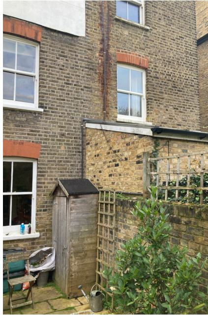
Existing rear view and neighbouring property.
