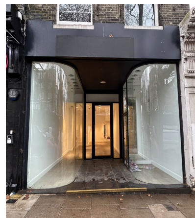
Existing shopfront view
