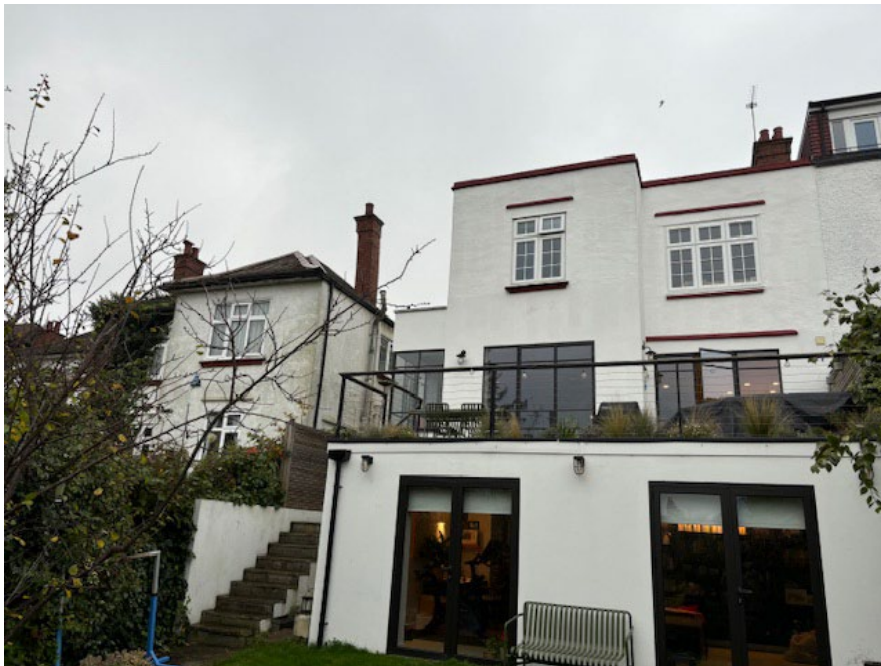
Rear view of No. 12 & 14.
