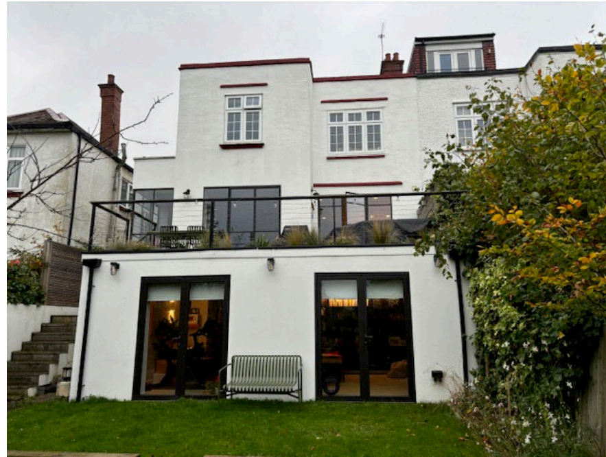
Rear view of No. 14 with existing extension granted in 2019
