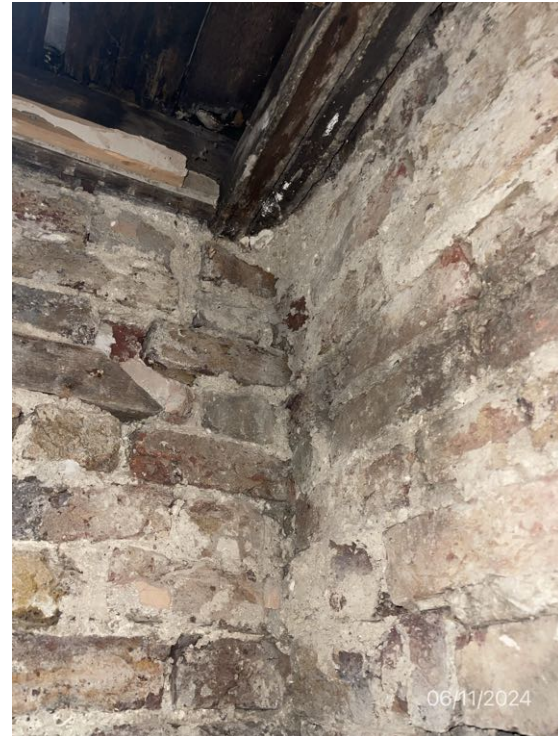
5. INTERIOR CLOSE UP VIEW
