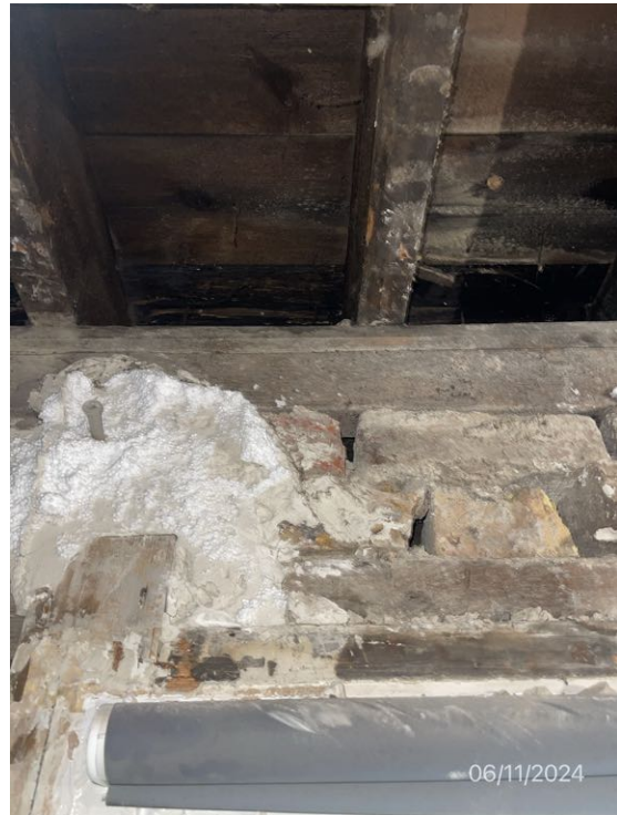
4. INTERIOR CLOSE UP VIEW
