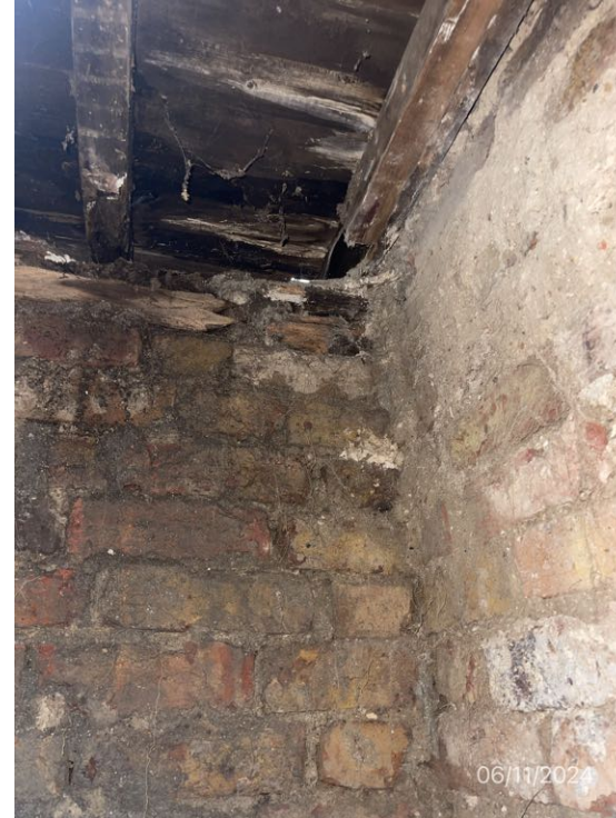
6. INTERIOR CLOSE UP VIEW
