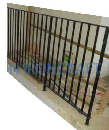
6(a).Steel Railings to balcony Painted black
