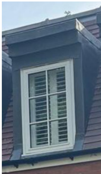
3. Leadwork: Lead Code 4 Roofing Lead Flashing Colour: Grey To match existing adjacent leadwork
