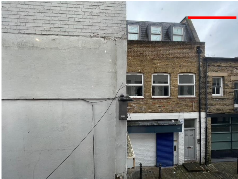
Figure 1 View from window 63, red line showing the height of the proposed development (including solar panels)
