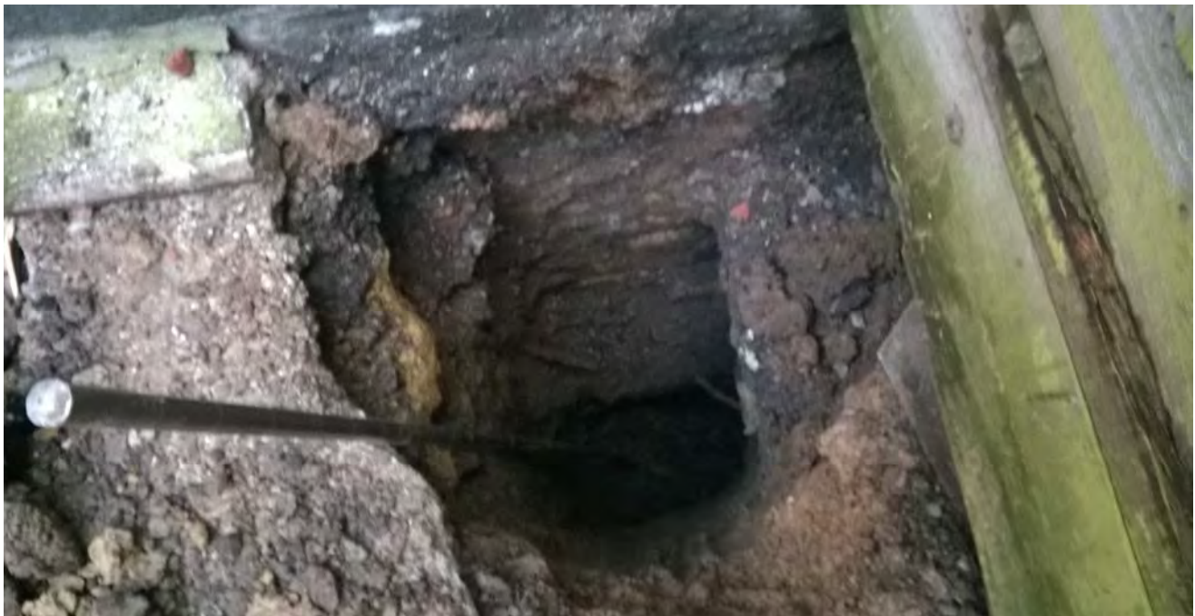
View into TP2 - looking southeast
