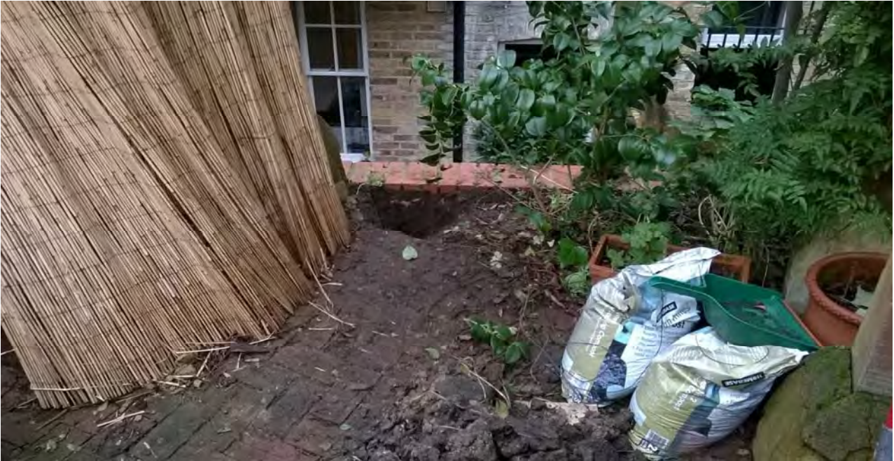
View of TP4 - looking northwest
