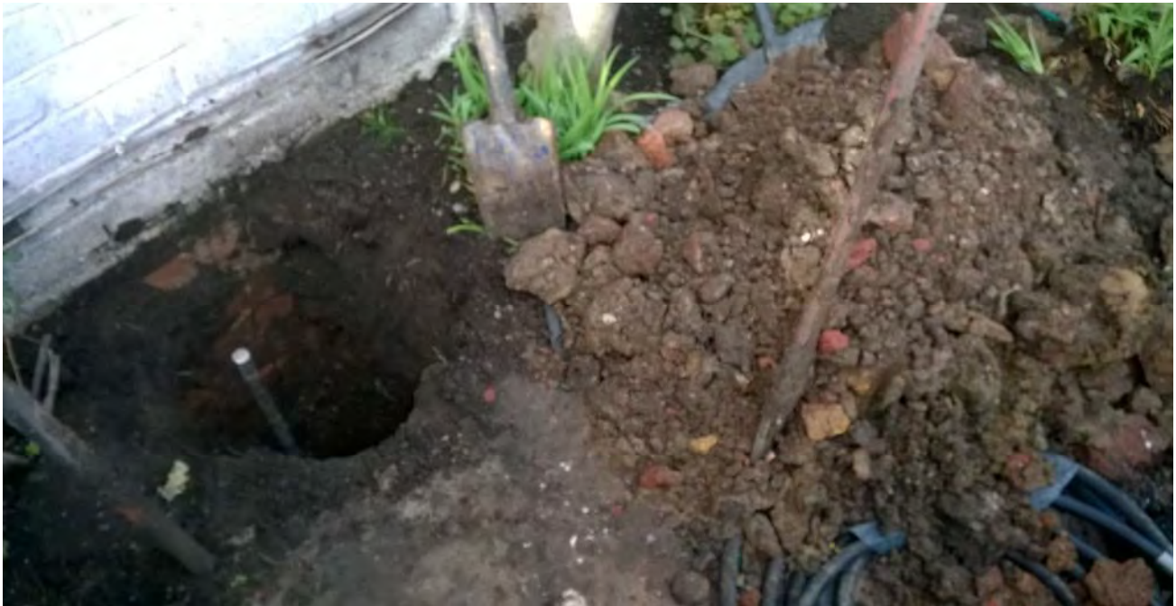
View of TP6 - looking northwest
