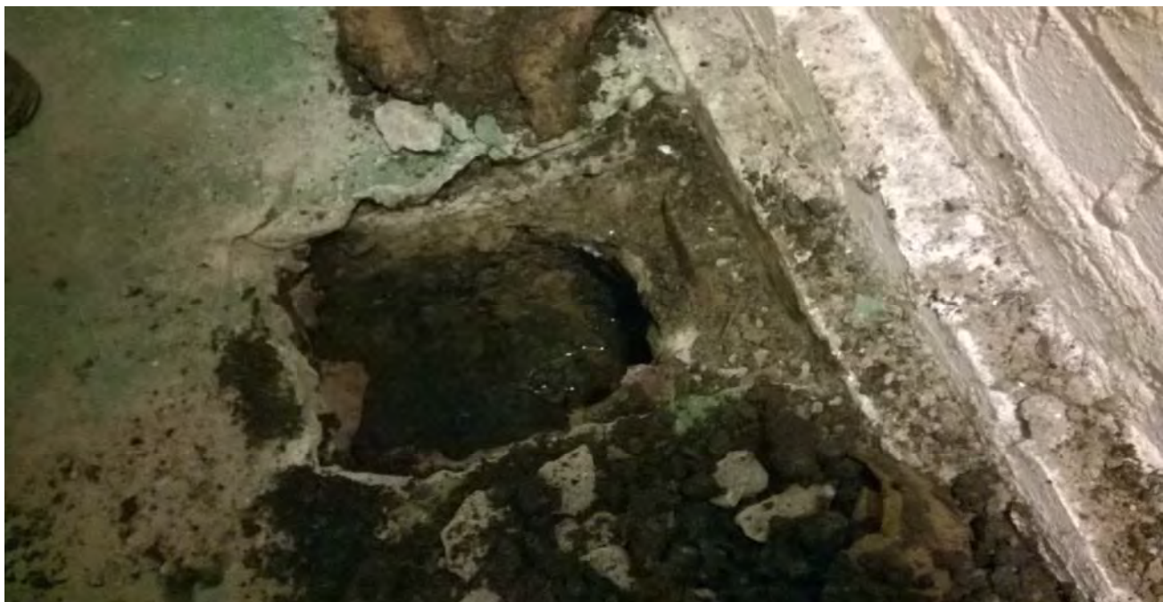
View into TP1 - looking southeast
