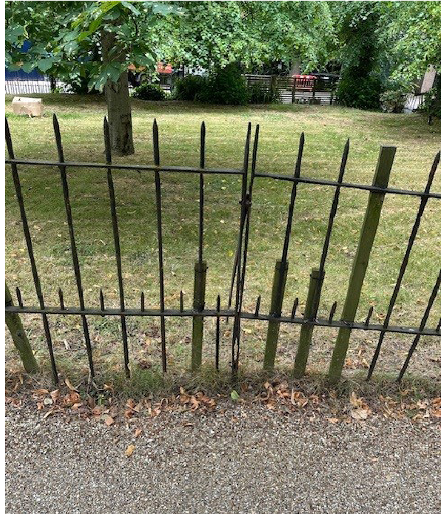
6. Panel with missing upright and dog rails
