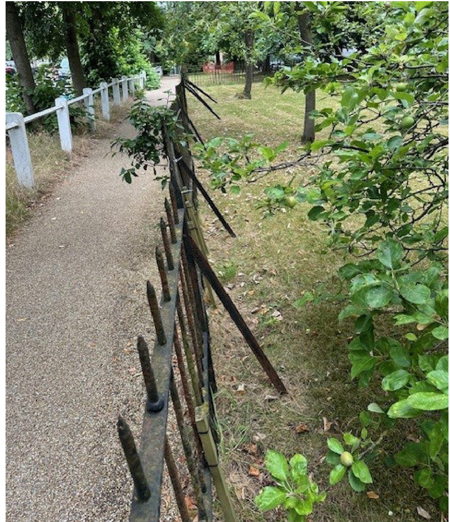
8. Remaining railings are bowed out and impede on to the adjacent footpath
