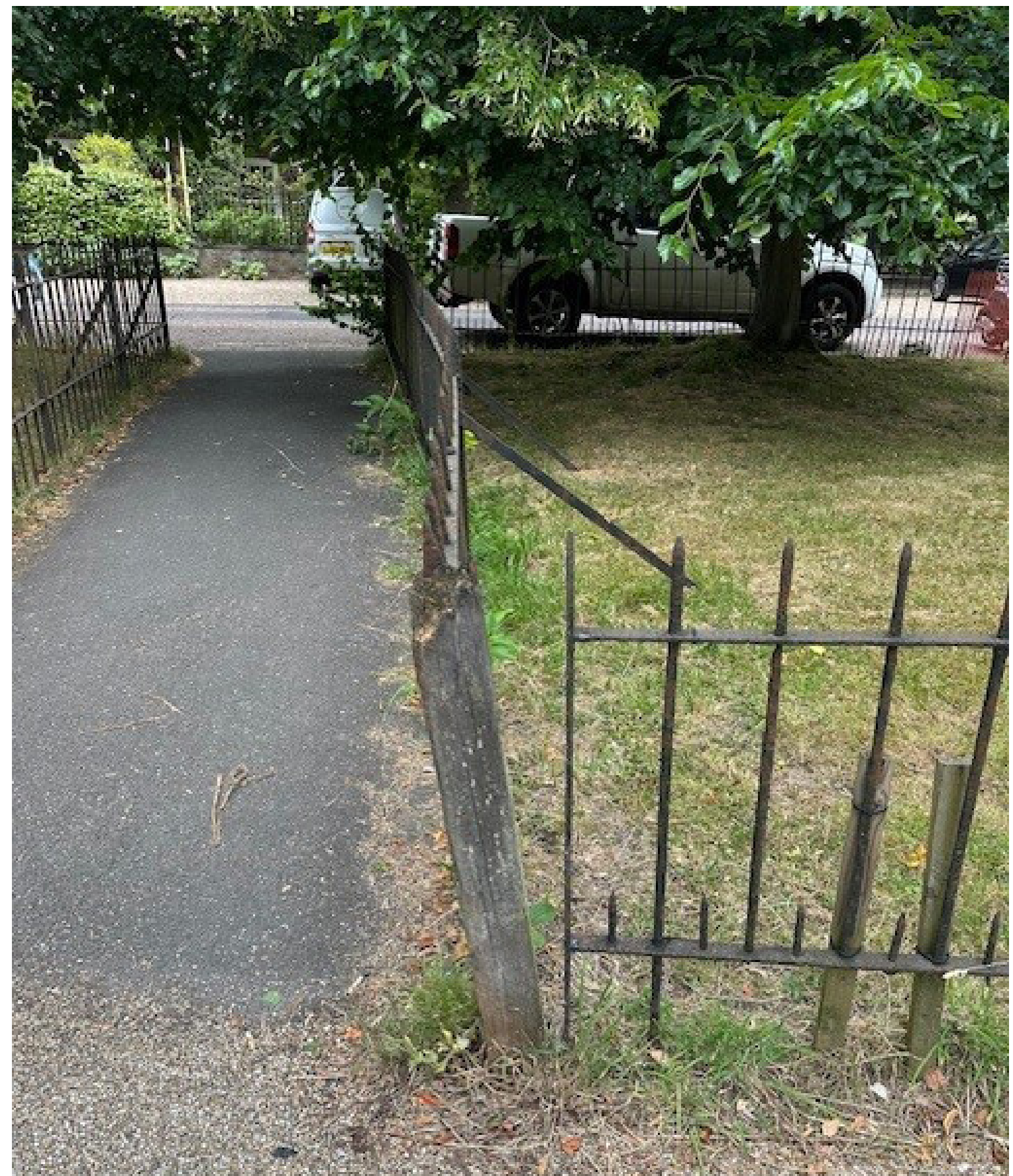
10. Small corner unit with missing upright and dog rails
