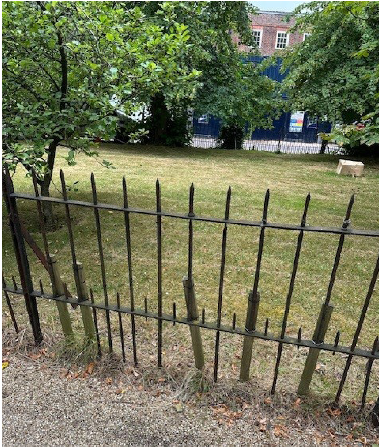
7. Panel with missing dog rails replaced
