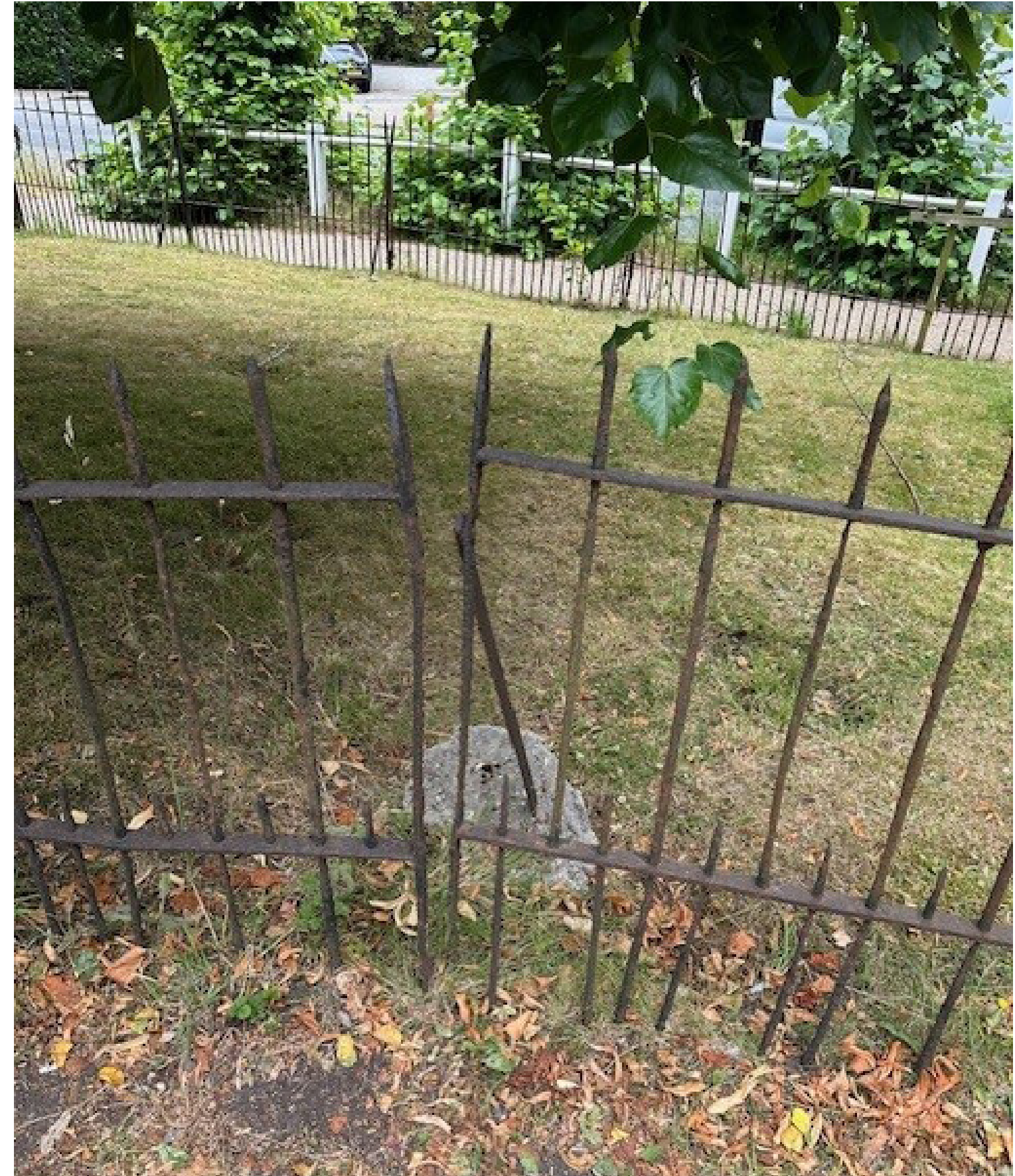
20. Broken connection between panels
