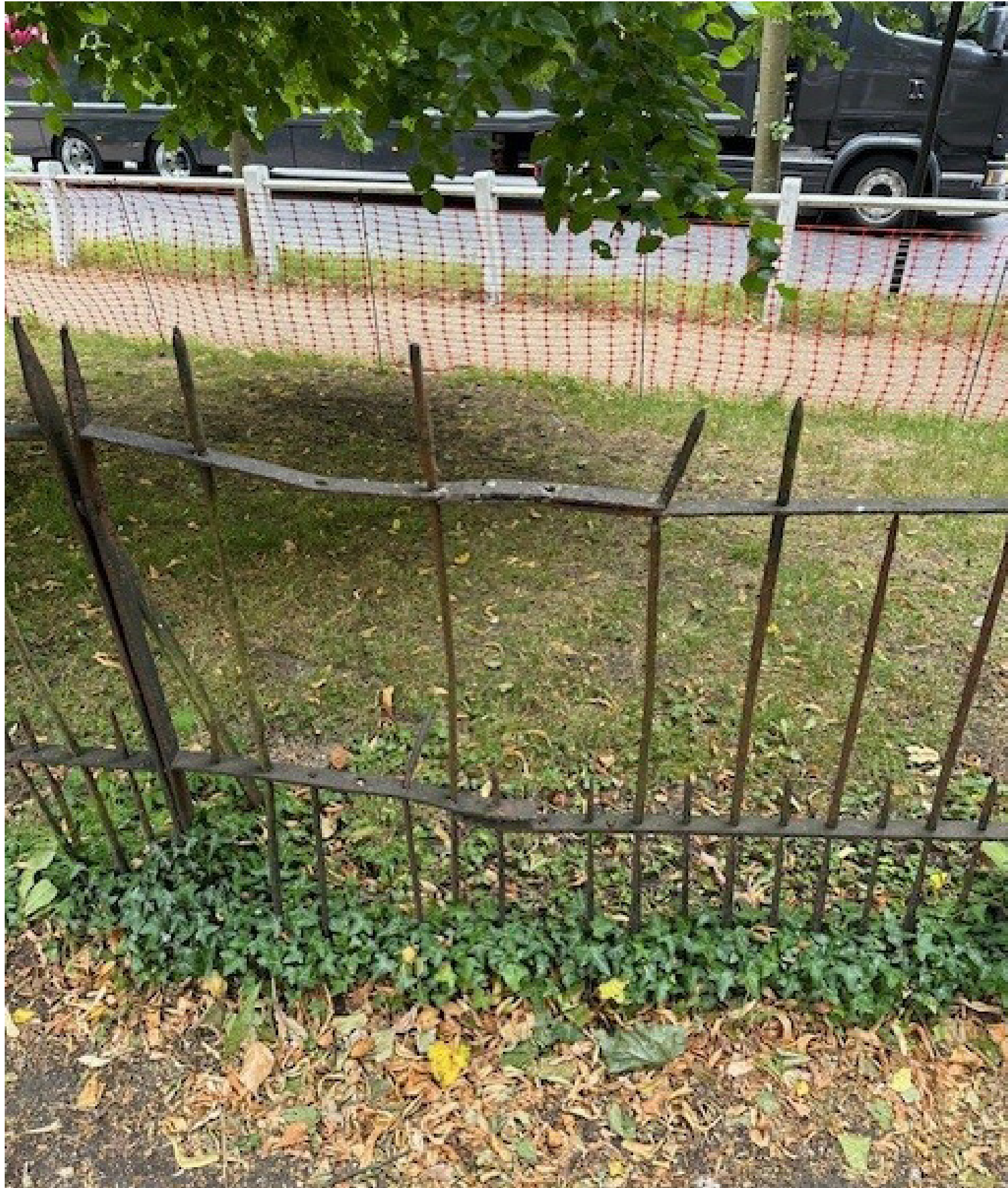
17. Panel With missing dog rails and upright
