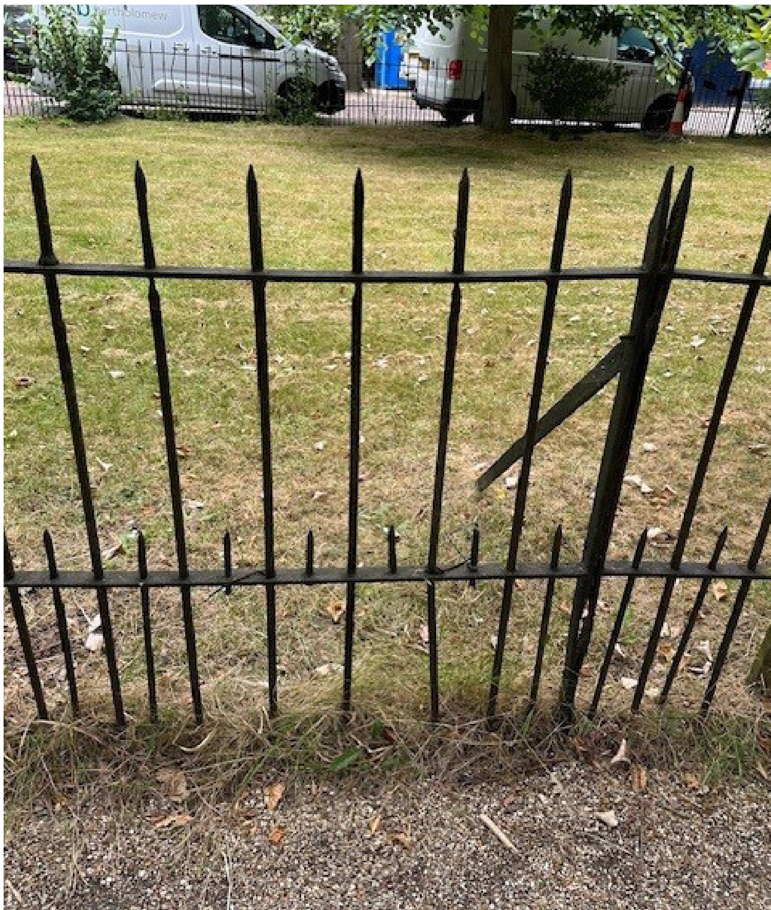
9. Connection is broken and bowing out
