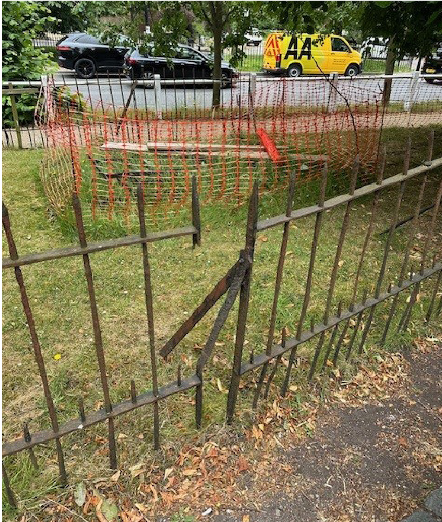
19. One panel missing end frame
