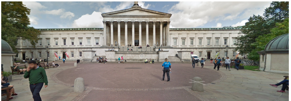
4. Internal view of Main Quad
