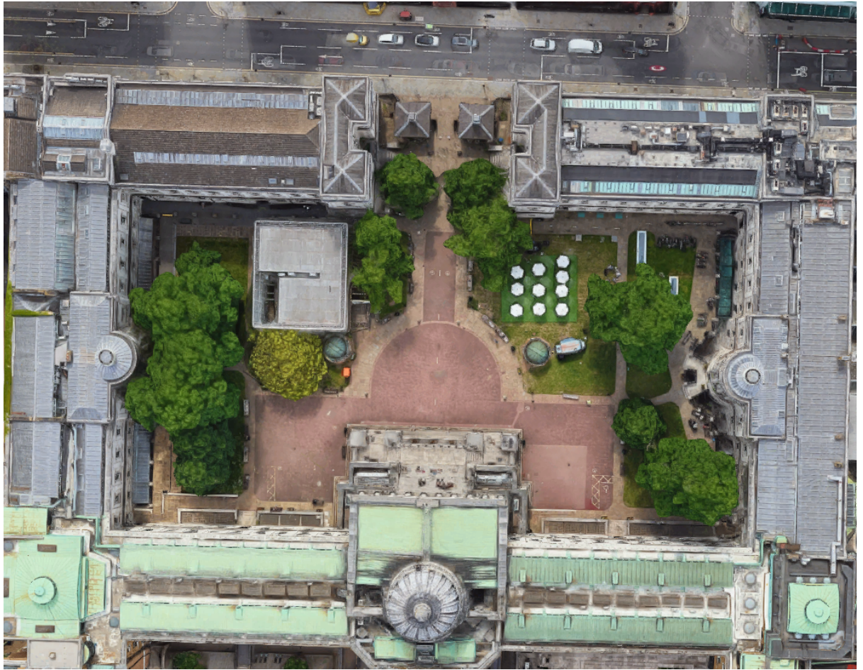
3. Top-down view of Main Quad and Wilkins roof
