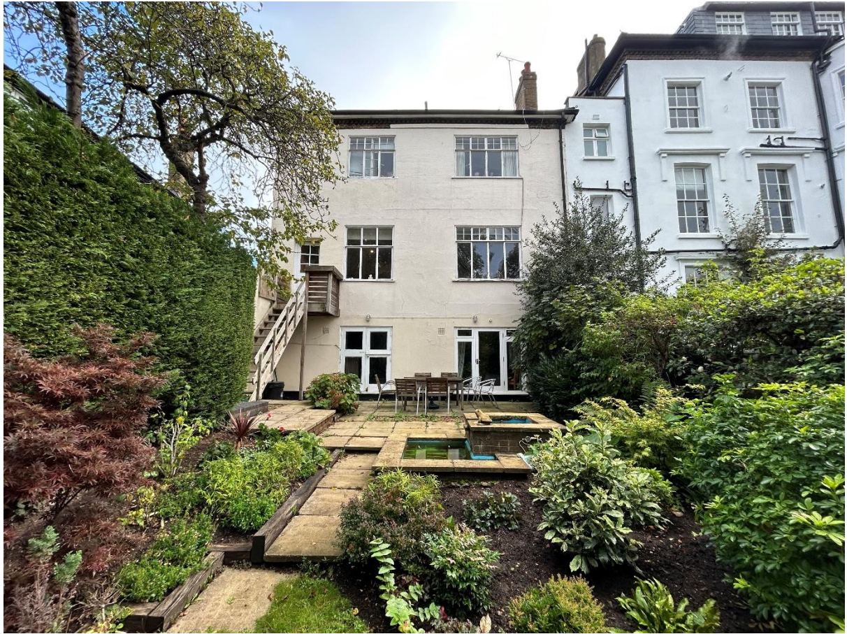
Figure 2. Rear of 40 Bramshill Gardens and adjoining property
