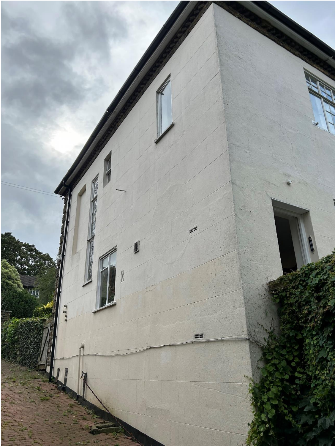
Figure 3. Side façade of 40 Bramshill Gardens
