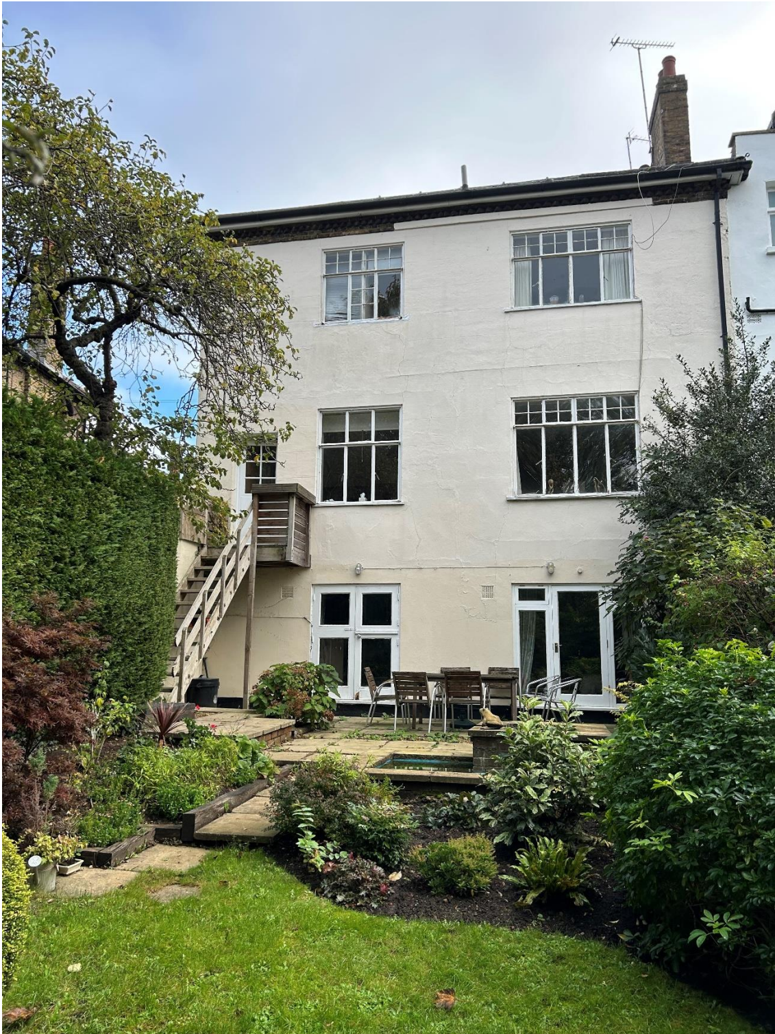
Figure 1. Existing glazing and door to the rear façade, with a notably shallow appearance to the glazing
