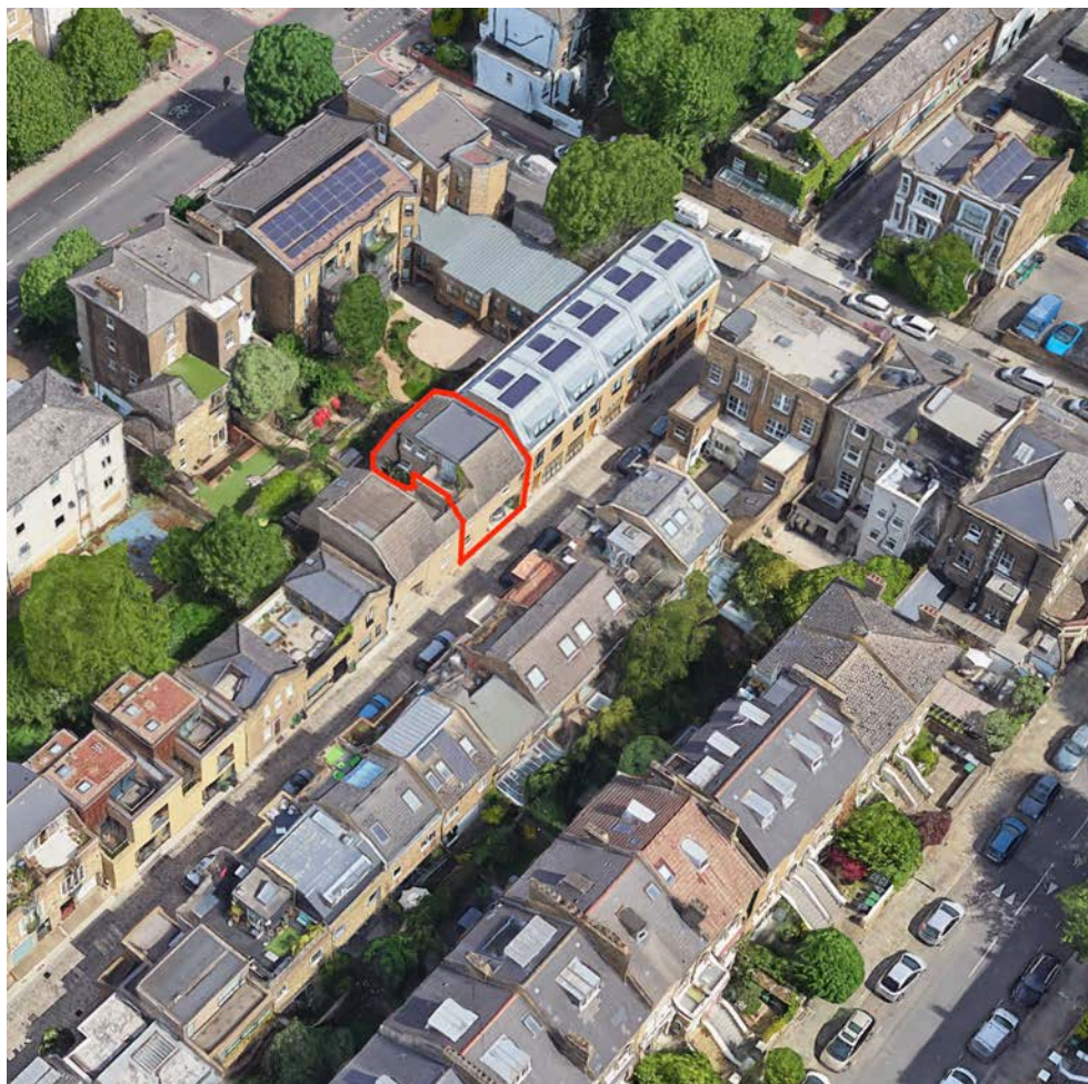
Aerial view of site
