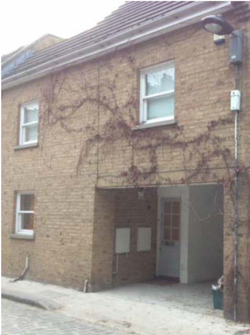
Application site, No. 103 Camden Mews.
