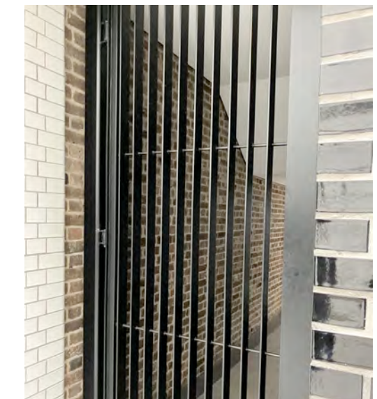
PRECEDENT IMAGE: METAL GATE: NARROW VERTICAL FINNS HELPS MAXIMISE LIGHT TRANSMISSION
