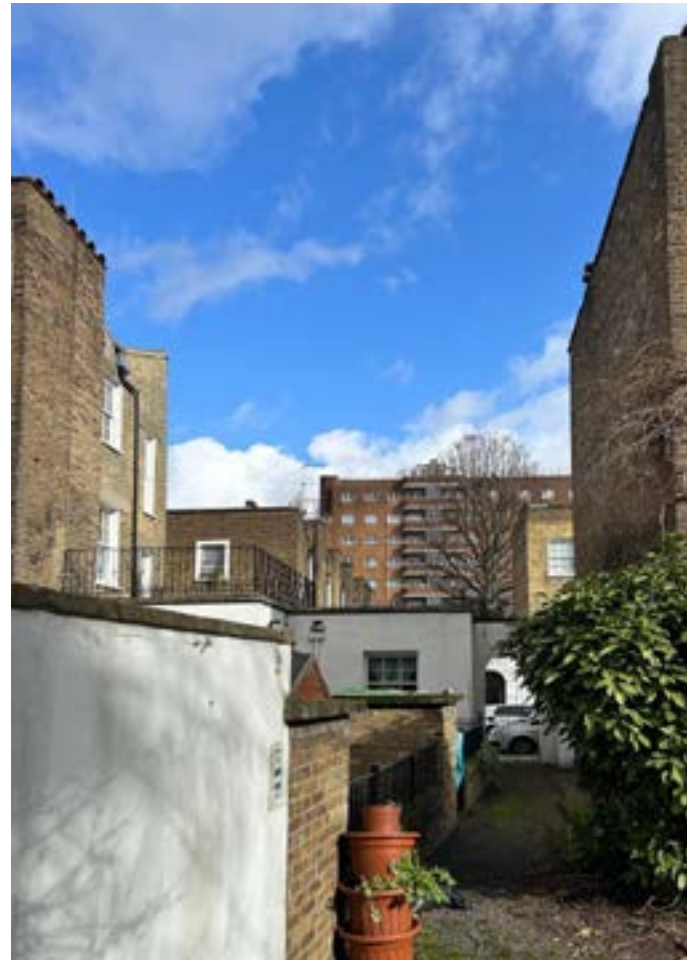
Figure 6.5 Existing view towards the rear of No. 26 Medburn Street along pathway from outside rear of No. 28 Medburn Street.
