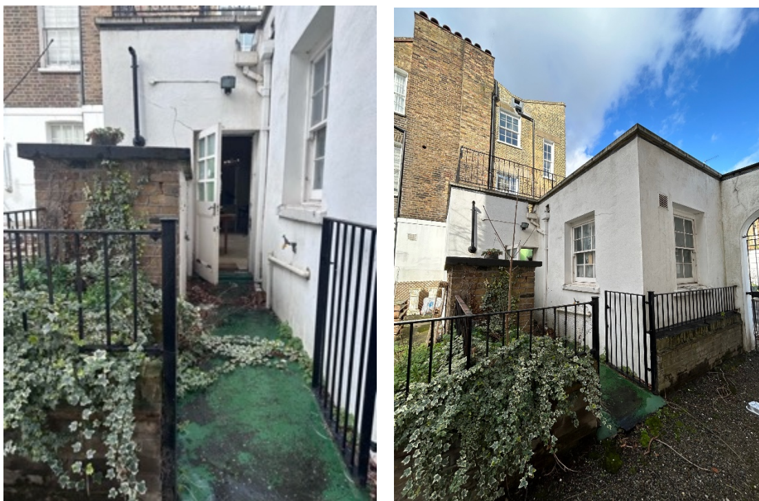
Photographs showing the existing passageway and view of the 1982 extension.
