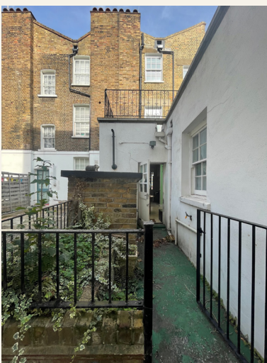
Figure 6: Photograph of rear view of existing external space and store.
