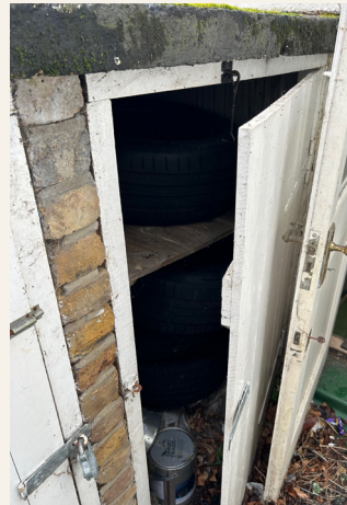
Fig.4: Photo of existing external store
