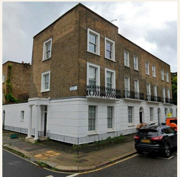
Fig. 1: External view of the property
