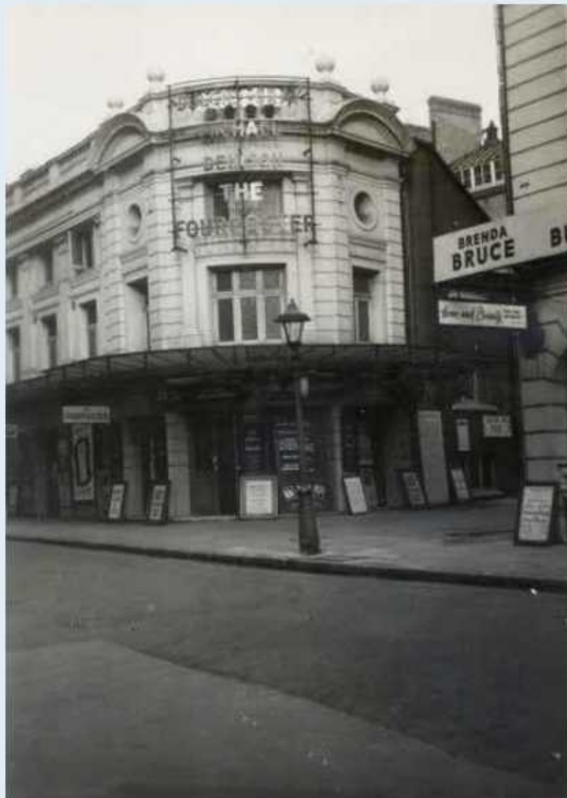
a) Photo of the exterior in c1950.
