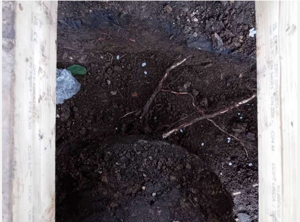
4 – 2x20mm horse chestnut roots severed within post hole P3.
