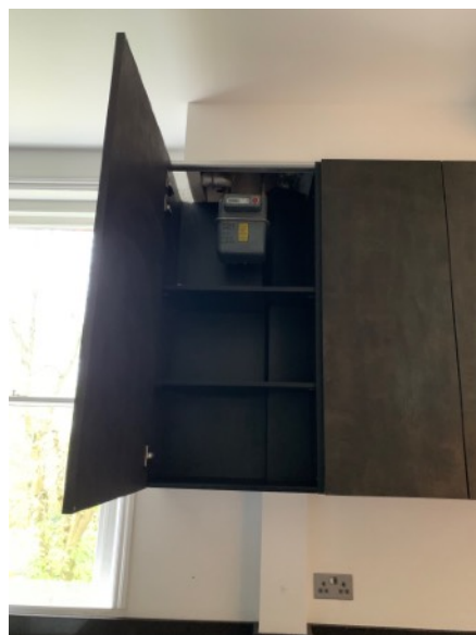
Fig 9 Gas meter to be moved to lower position removing duct for pipe.
