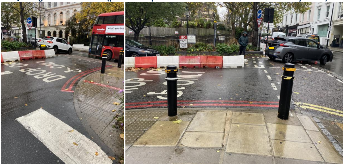
Figure 8 – Queuing from Pond Street (photo from previous site visit on 15 November 2022 by Evoke)
