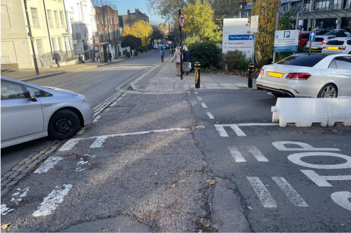
Figure 6 – Queuing back on to Pond Street
