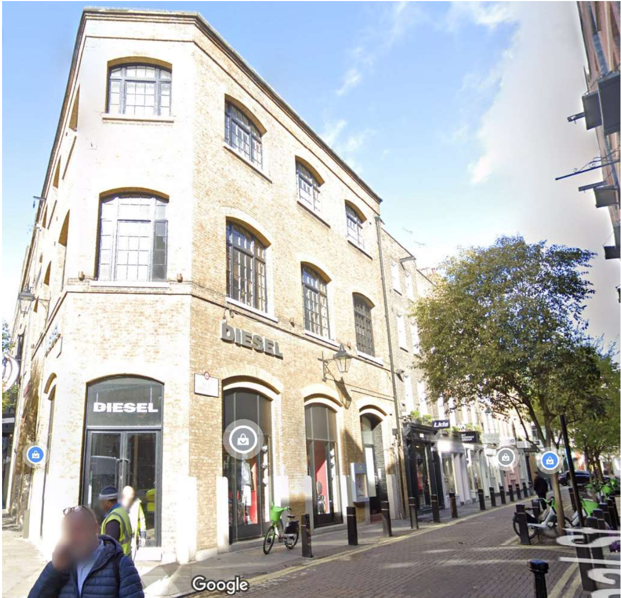
Existing building – Neal Street elevation
