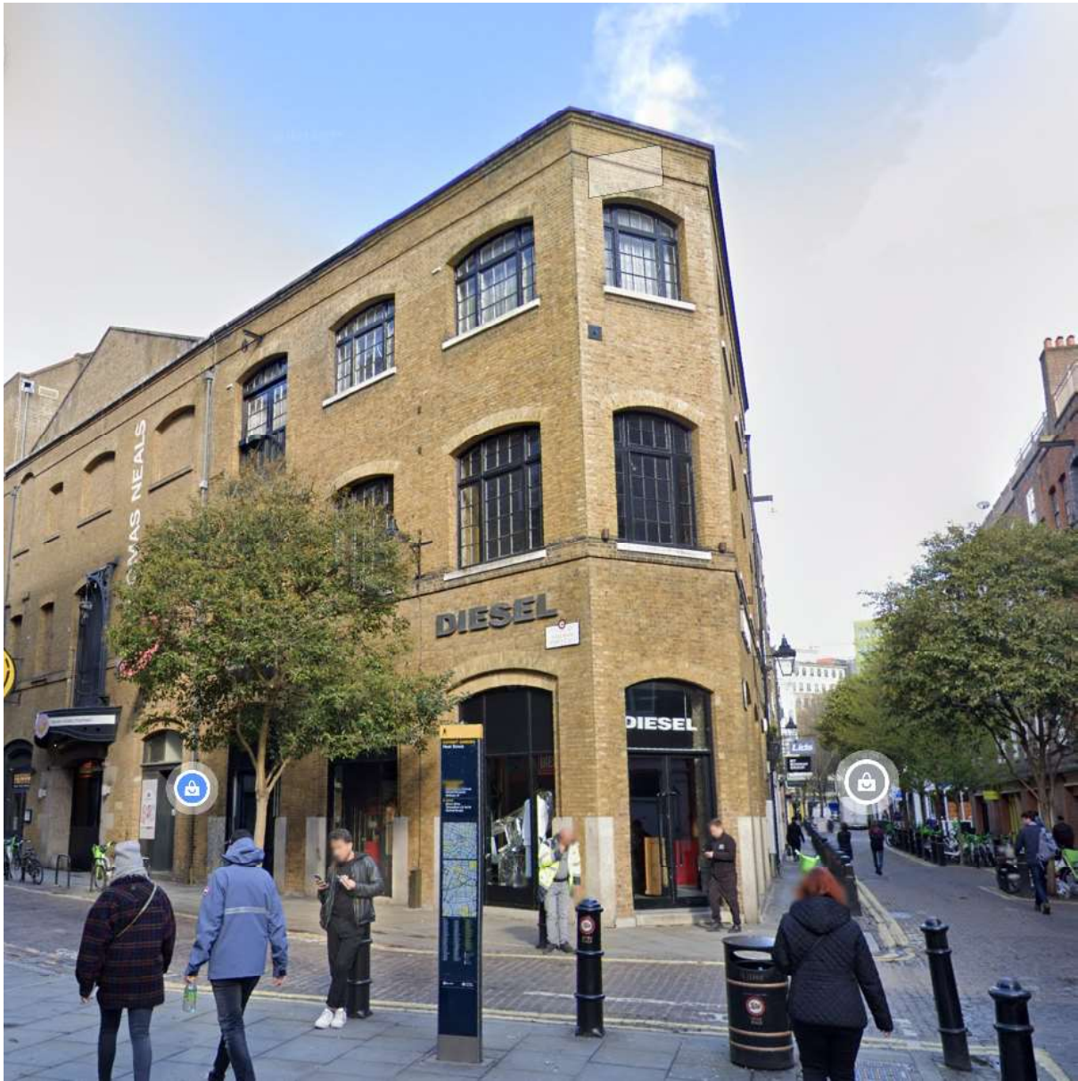
Existing building with existing signage
