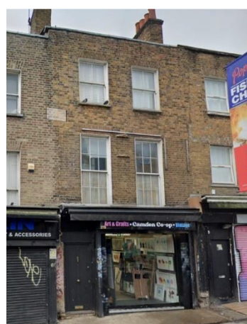
Figure 5.12: 279 Camden High Street
