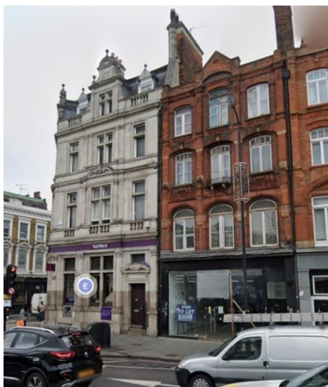
Figure 5.1: 166 / 169 Camden High Street
