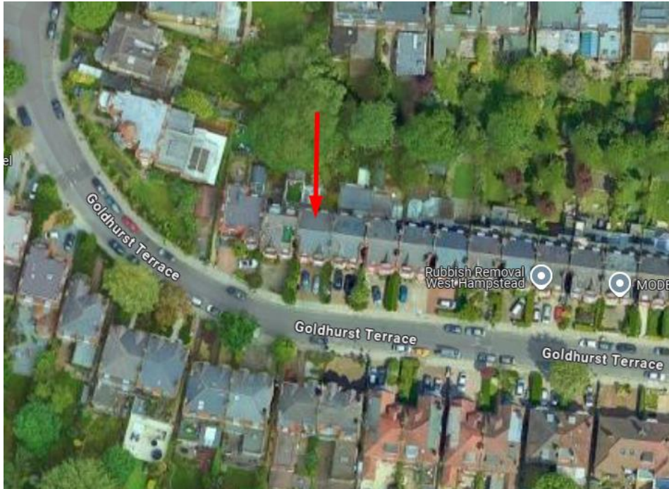
Figure 1 Aerial view of 188 Goldhurst Terrace
