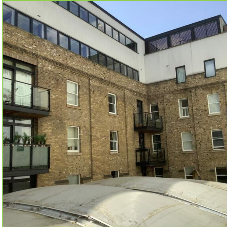
Figure 8.8: Courtyard North-east facing elevation showing masonry and render system.
