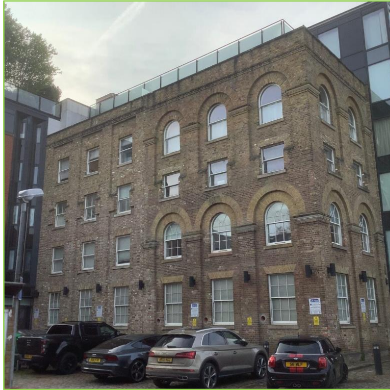
Figure 8.4: North-west Elevation showing original Victorian façade.
