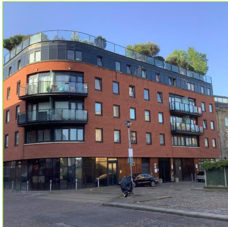
Figure 8.5: North facing Elevation showing masonry, aluminium spandrels and timber cladding at ground level.
