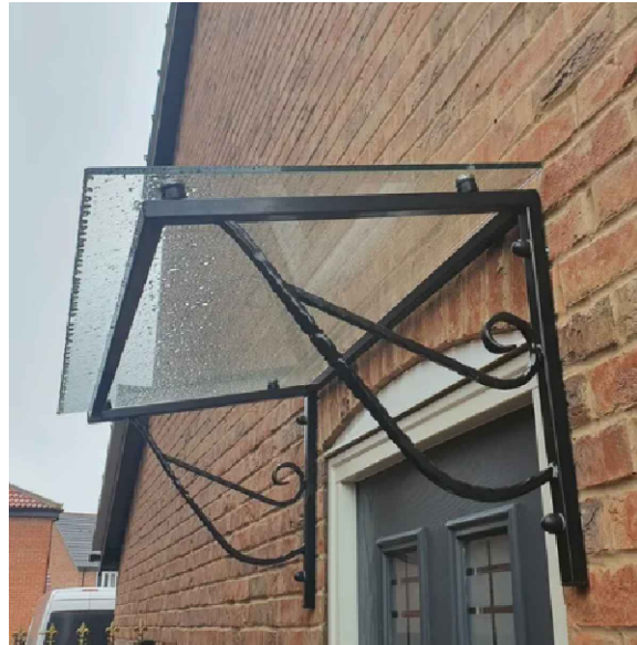
Steel Glass Canopy
