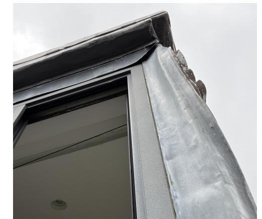
View of the applicant's dormer window and close up of dormer from outside showing lead cladding and traditional overhang
