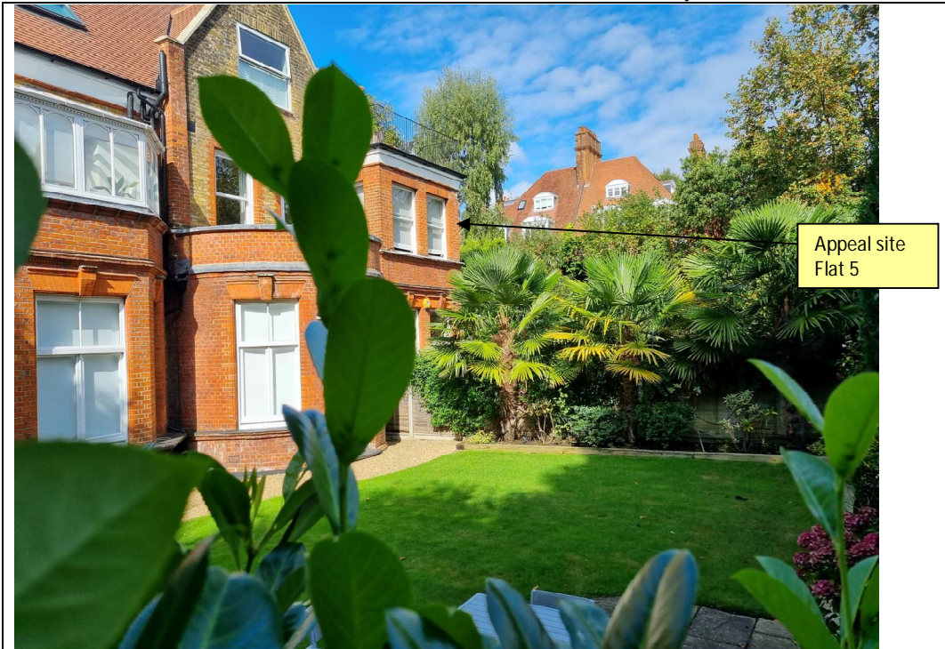
View of the rear north-east facing elevation to No.1 Lyndhurst Road looking onto the rear gardens to the ground floor flats. The garden is split into two. In the foreground is the garden to Flat 1. Behind the extensive foliage in the background is the garden to Flat 2 separated by a wooden fence (hidden by the foliage). In the far distance the roofs to Nos. 11 & 13 Akenside Road can be seen. Flat 5, the appeal site (marked) is located on the far corner at first floor level.
