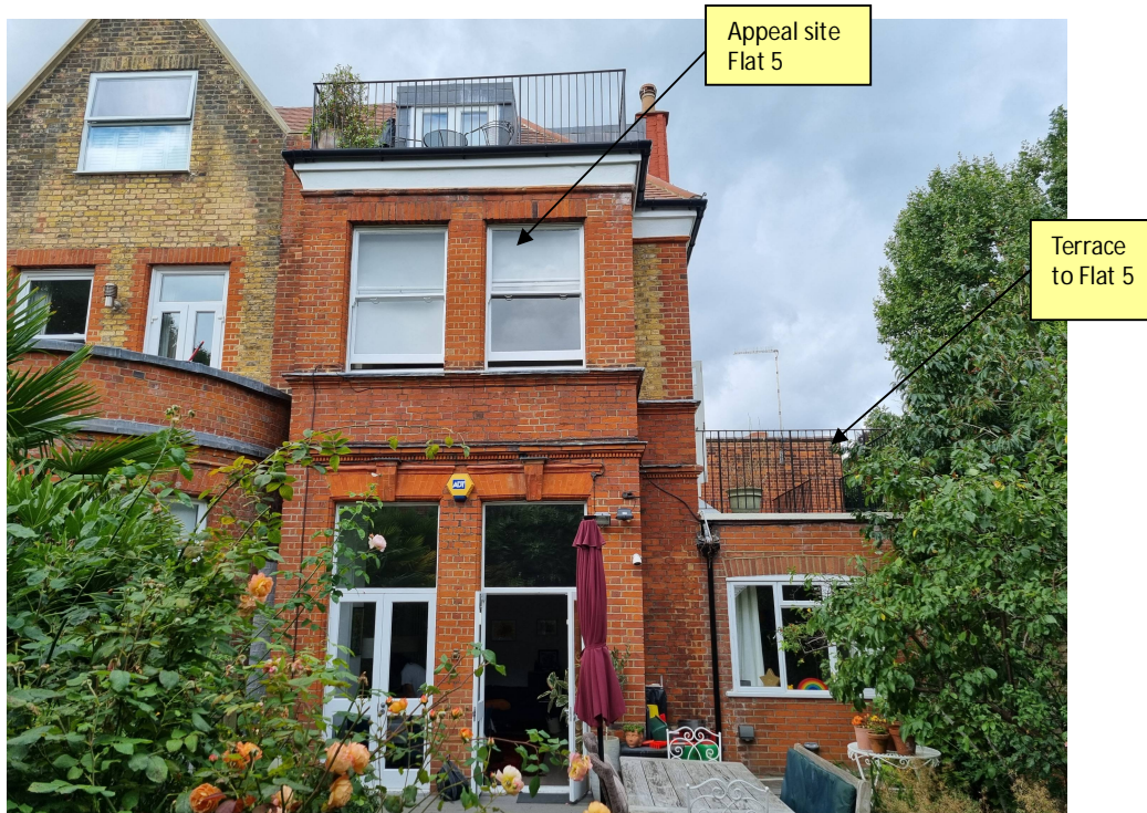
View of part of the rear north east facing elevation as seen from the garden to the ground floor flat, Flat 2. The proposed location of the conservatory is on the terrace above the single storey side extension seen on the right. The terrace (as marked on the photo) to Flat 5 is located in the most concealed part of 1 Lyndhurst Gdns.
