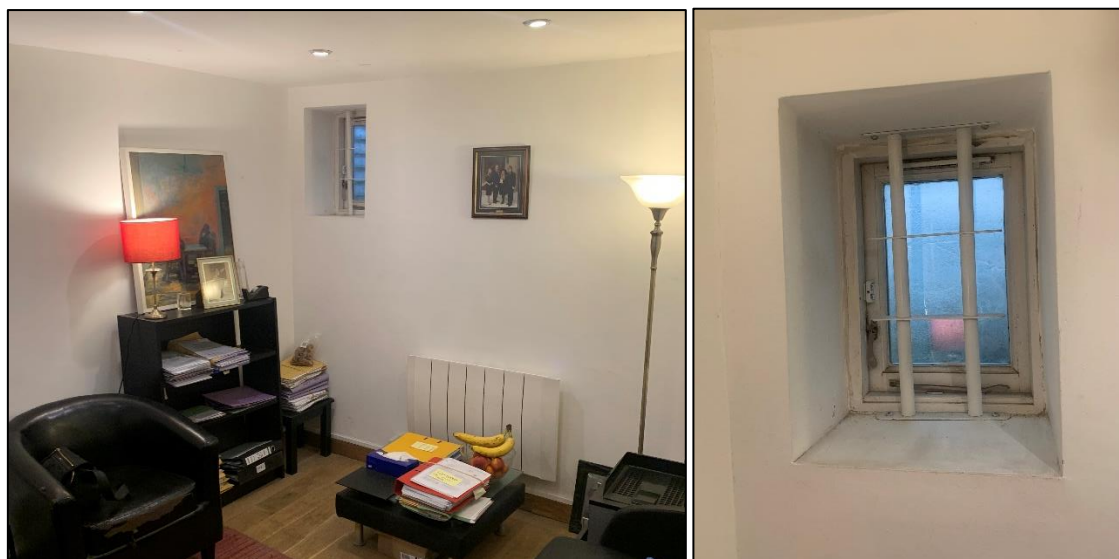
Fig 1. Existing rear basement room (left) and basement window (right).
