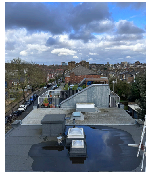
View of existing roof top
