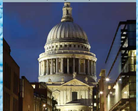
St Pauls Cathedral Damp Proofing & Tanking works by Kenwood Plc
