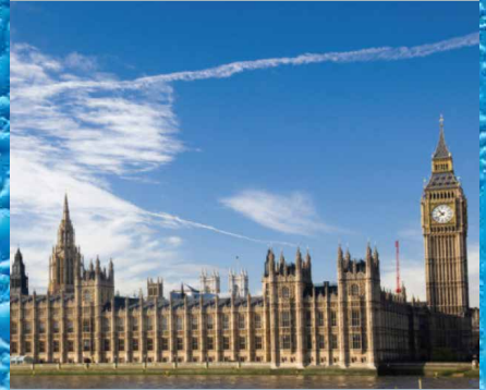
Parliamentary Works Damp Proofing & Tanking by Kenwood Plc
