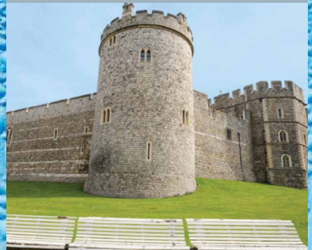
Windsor Castle Structural Waterproofing works by Kenwood Plc
