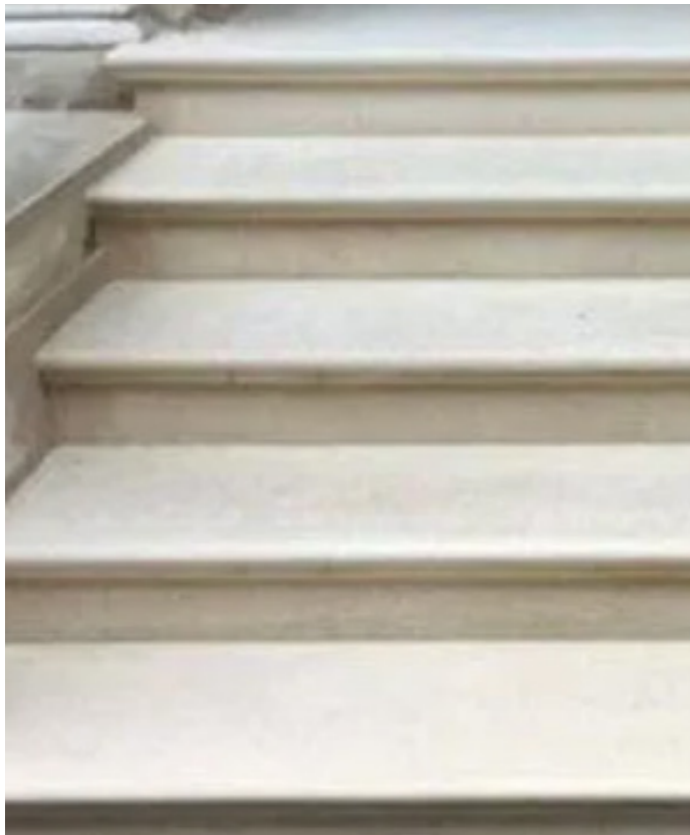
Portland Stone cladding for the front and back steps
