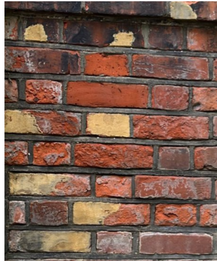
Smooth reclaimed red brick for the wall and balustrade (material matching existing)
