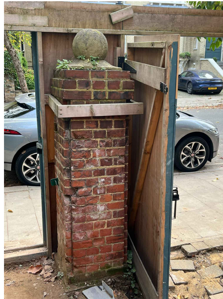
Photograph of existing pillar to be reconstructed
