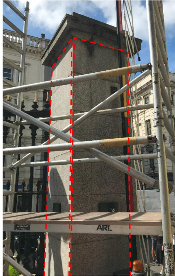
**Plate 1:** Photograph of the gate pier showing the two faces scanned during the GPR survey (highlighted in red).
