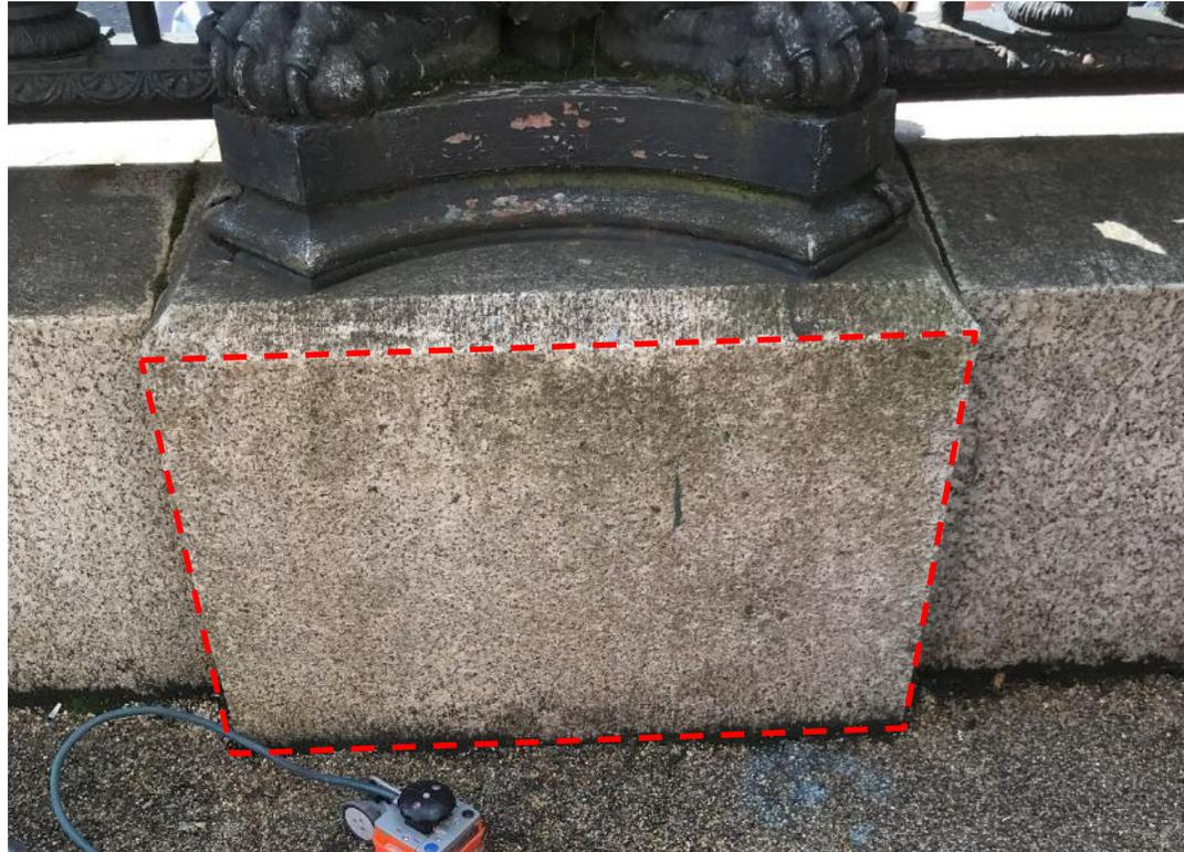
**Plate 2:** Photograph of the granite support wall showing the area scanned during the GPR survey (highlighted in red).
