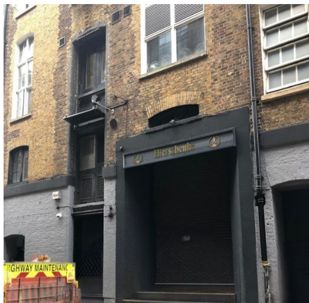
Figure 3 – Shelton Street Frontage
