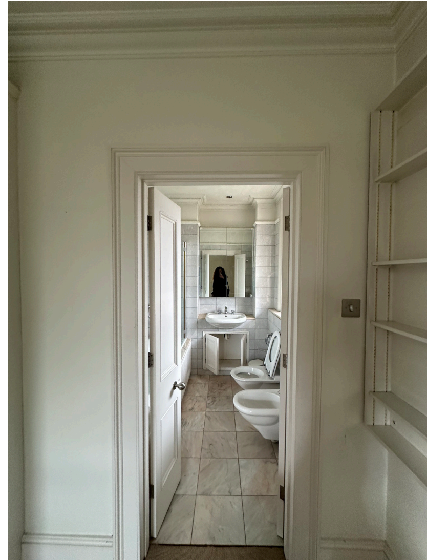
Existing second floor bathroom door
