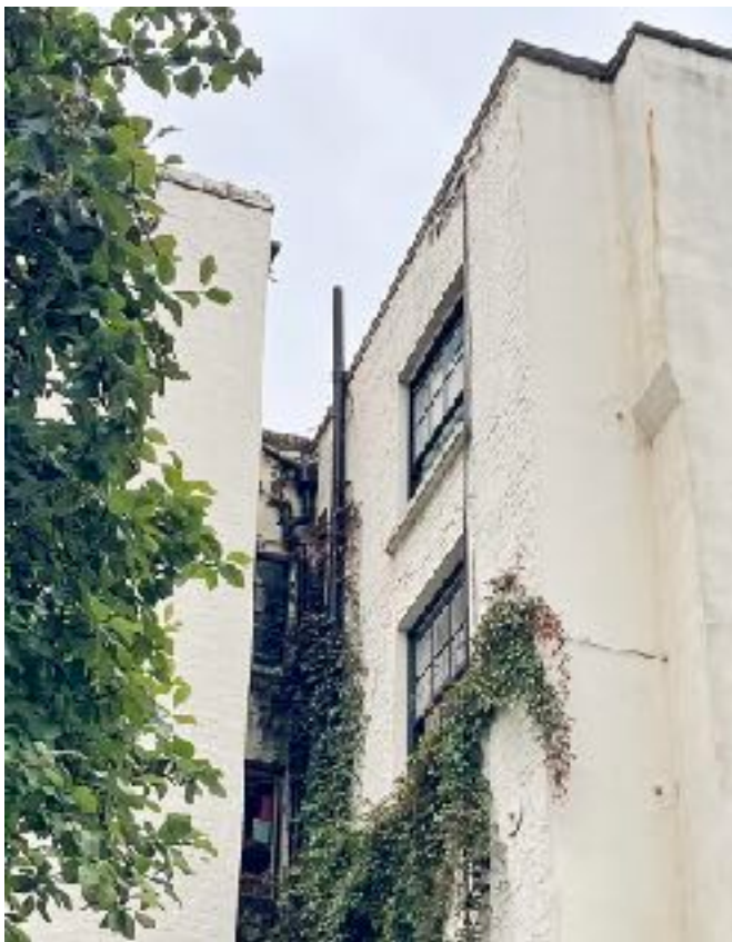
Rear Elevations Bathroom vent Location
