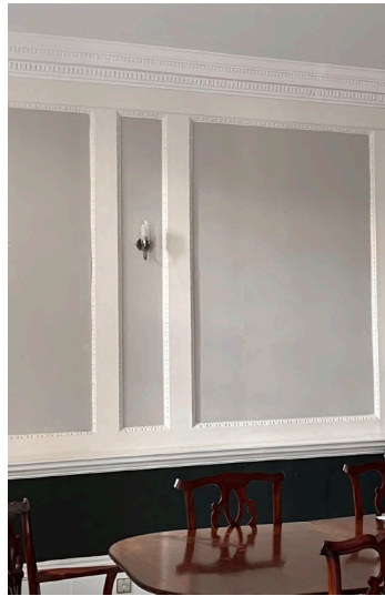
Existing Wall Panels on Ground Floor
