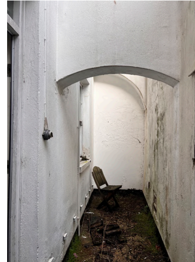
Basement Rear External Light Well
