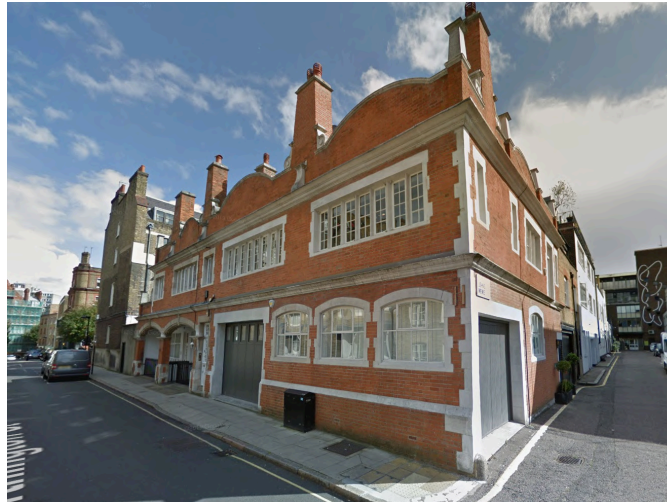
2. 13 Northington Street REF: Google Maps
