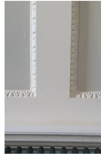
Detail of Existing Wall Panels on Ground Floor
