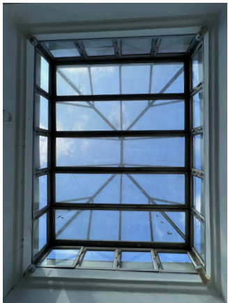
Existing Roof Lantern
