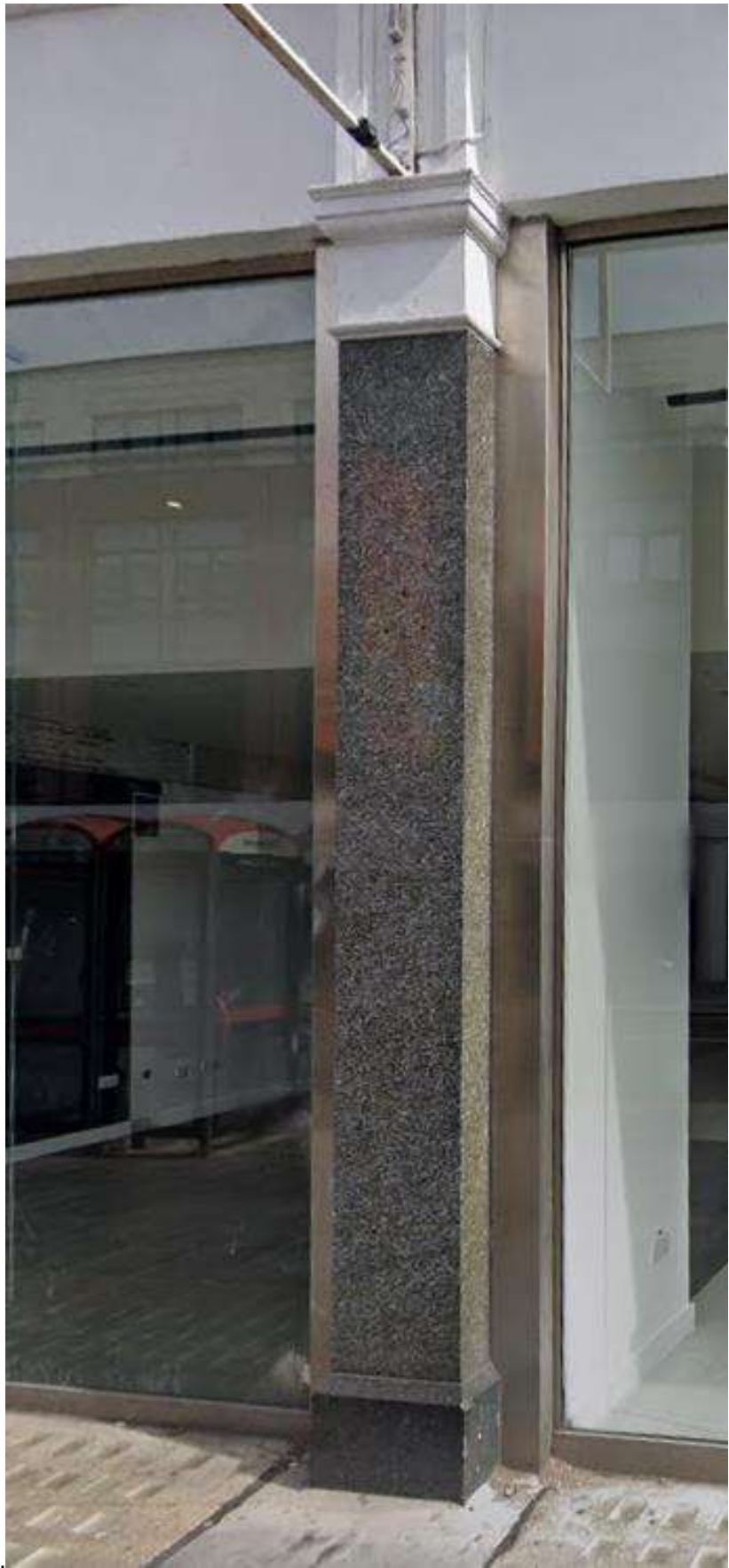
Figure 31: Detail of the stone panels at ground floor level (Tottenham Court Road)
