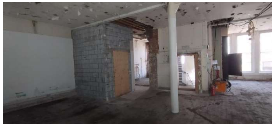
Figure 7: Concrete blocks shaft in Building 2, first floor
