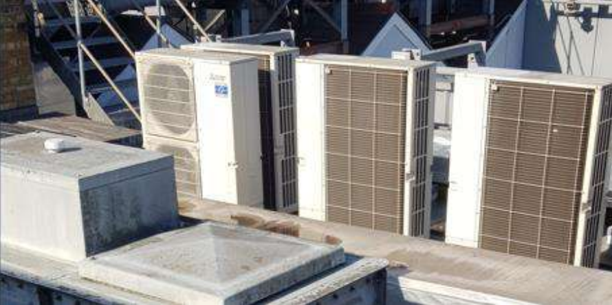
Figure 22: Individual AHU on the roof
