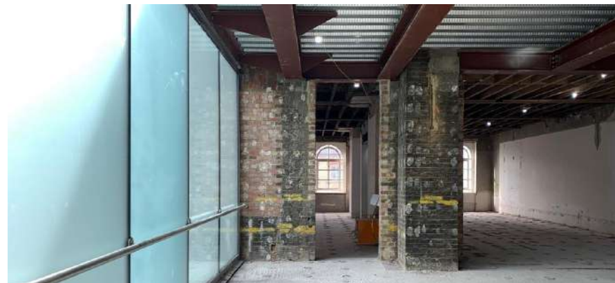
Figure 11: Metal deck in Building 5 (Second floor level)
