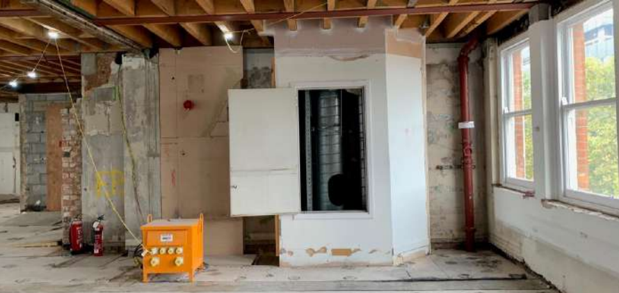
Figure 25: Plasterboard in the riser of Building 2, second floor
