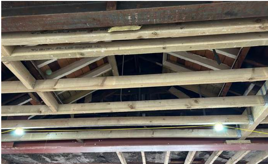
Figure 19: 3rd floor timber & steel roof structure
