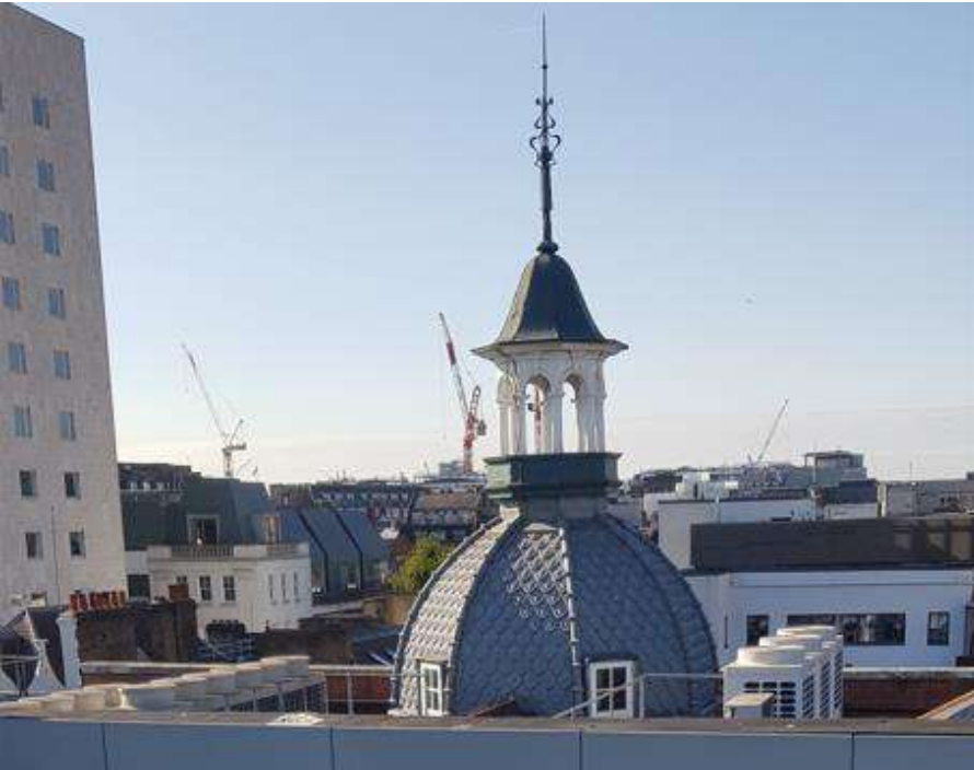
Figure 20: Timber-framed cupola topping Building 1
