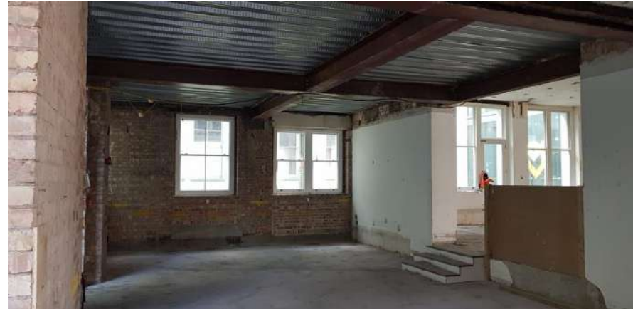
Figure 9: 1-3 Alfred Place (Building 2): steel beams and metal deck
