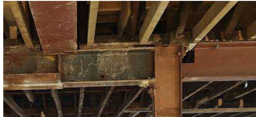
Figure 4: Photo of unorthodox steel detailing in steel grillage. Key issues include lack of appropriate stiffeners and end plates to beams & top plate to columns.
