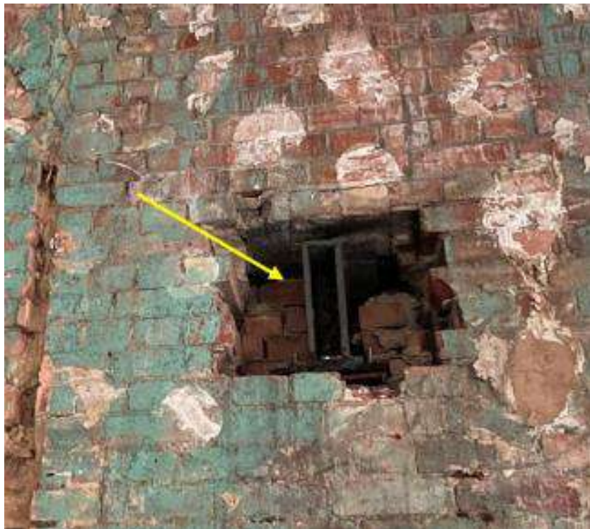
Figure 3: Penetration through external wall of building 3.
