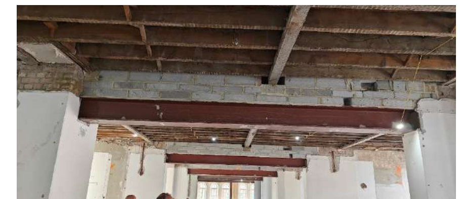
Figure 2: Openings through load bearing walls in Building 1.
