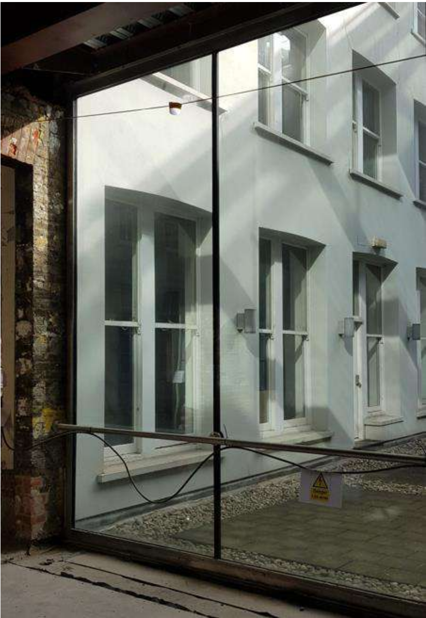
Figure 17: Glass partition between Building 5 and the courtyard
