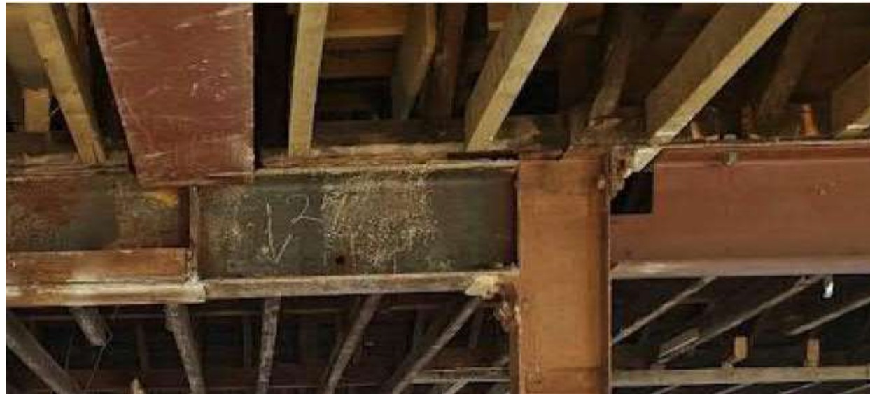
Figure 5.3.2: Unorthodox steel detailing in steel grillage in 220-226 Tottenham Court Road. Key issues include lack of appropriate stiffeners and end plates to beams & top plate to columns.
