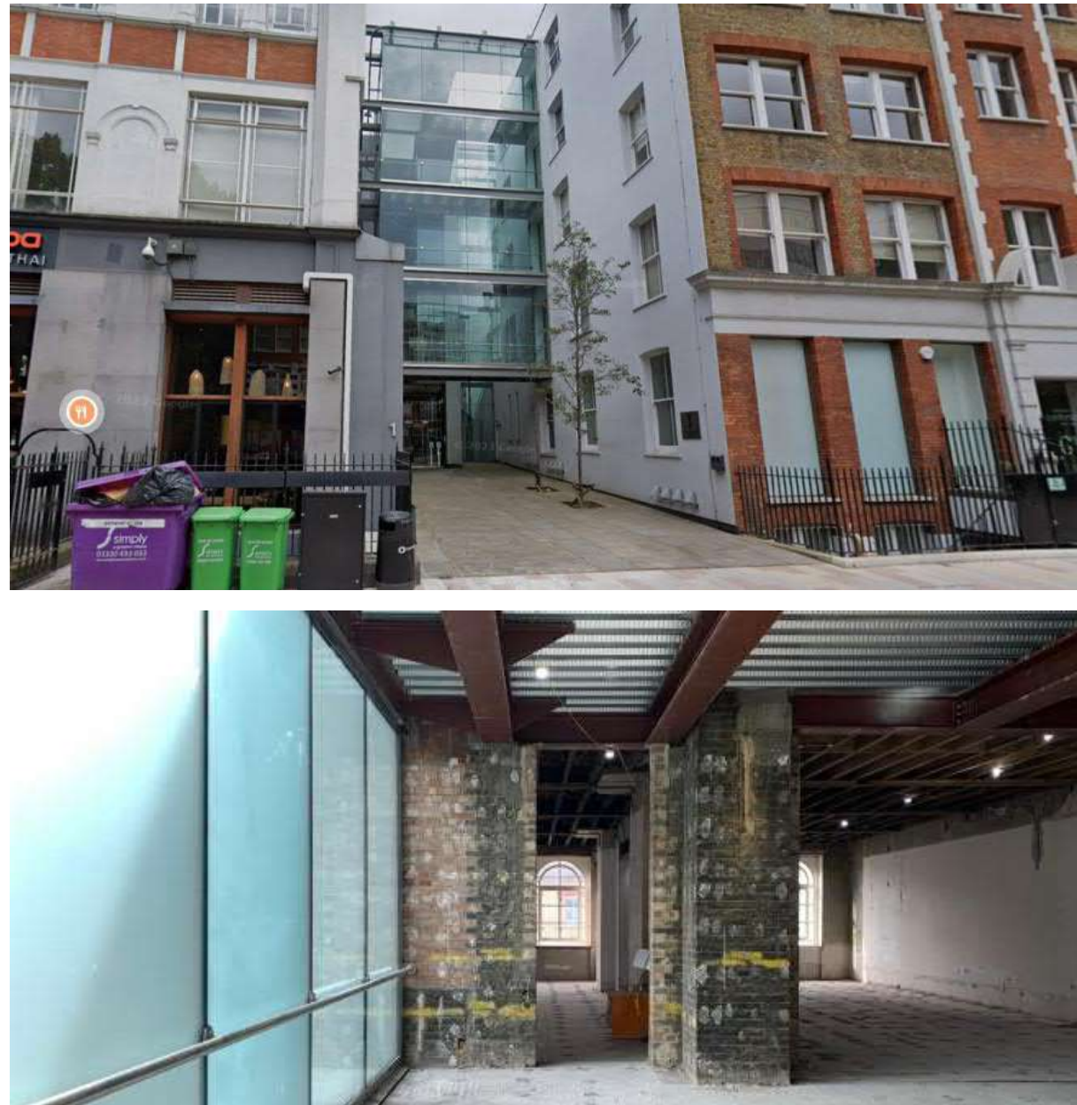
Figure 5.3.4: Steel structure of the link building (first image) and internal image of steel and metal deck system (second image).
