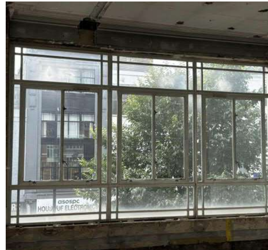
Figure 5.4.2: steel frame windows to Tottenham Court Road and Store Street.
