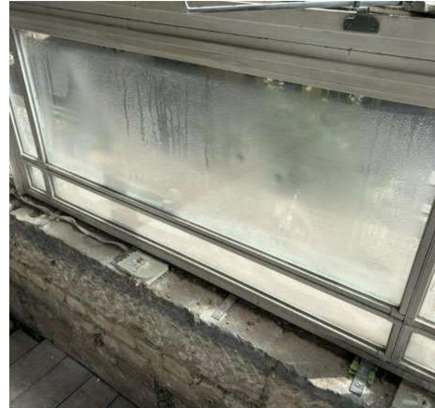
Figure 5.4.4: evidence of failure of DGUs.
