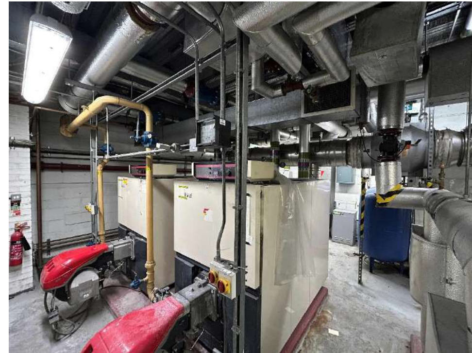
Figure 4.1.2: existing natural gas boilers at basement (via project team site visit).
