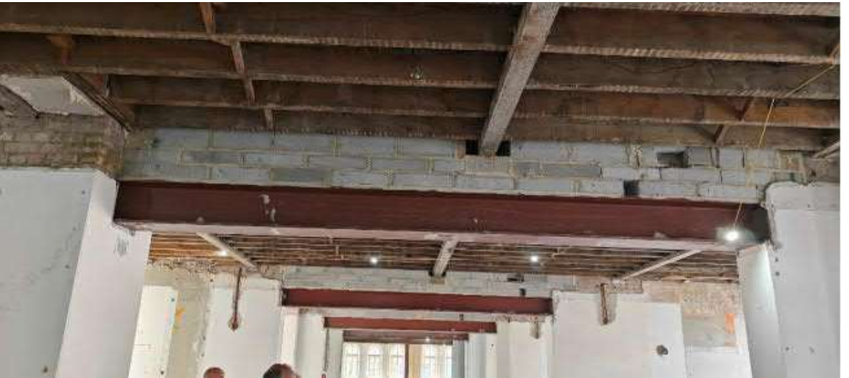
Figure 5.3.1: opening & load-bearing walls in 220-226 Tottenham Court Road.
