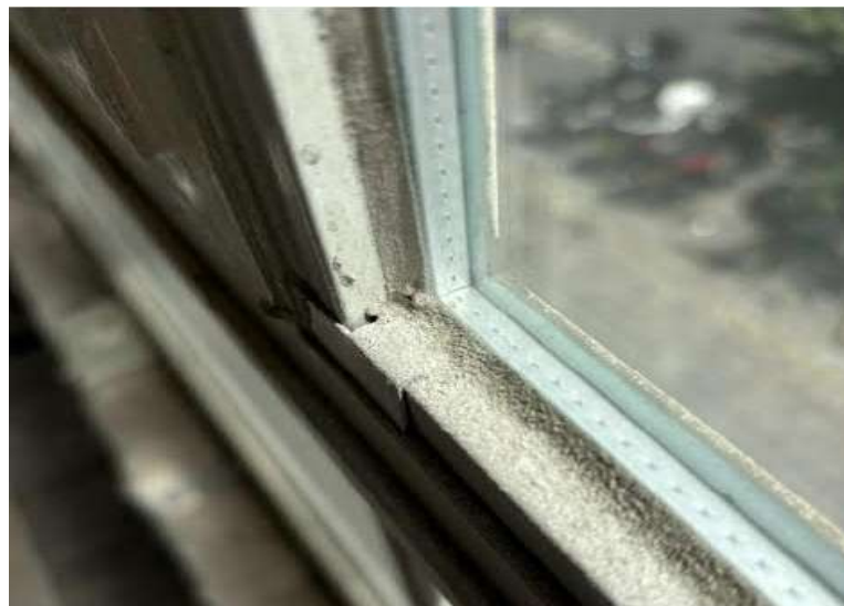
Figure 5.4.1: DGU glazing to Tottenham Court Road and Store Street elevations.
