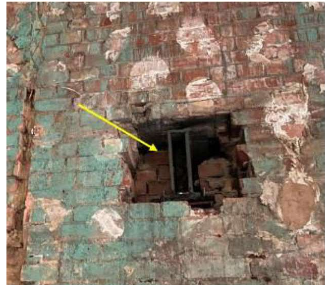
Figure 5.3.3: penetration through external wall of 22 Store Street.
