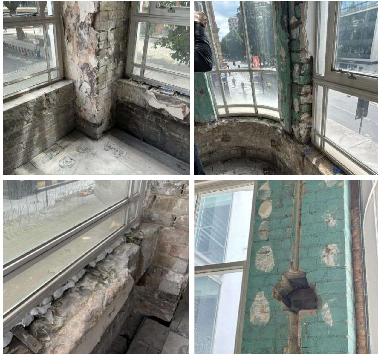
Figure 5.4.5: condition of brick piers and façade/glazing interfaces.
