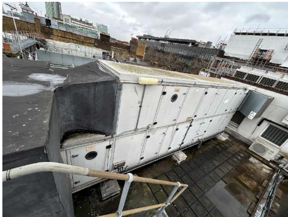
Figure 4.1.1: AHUs at roof level (via project team site visit).
