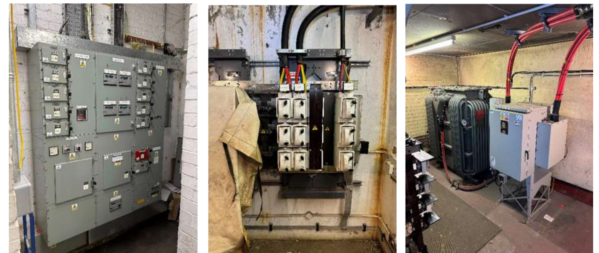
Figure 4.1.3: typical images of age, state and condition of existing electrical equipment including switchgear and transformers (via project team site visit).
