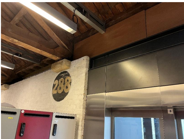
Figure 19 Lift panelling interacting with brickwork (private access space)
