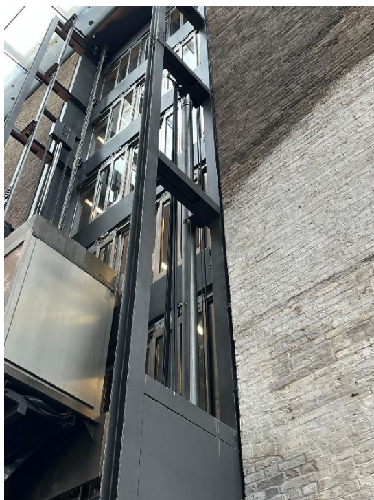
Figure 16 Lift steelwork adjacent the brickwork.
