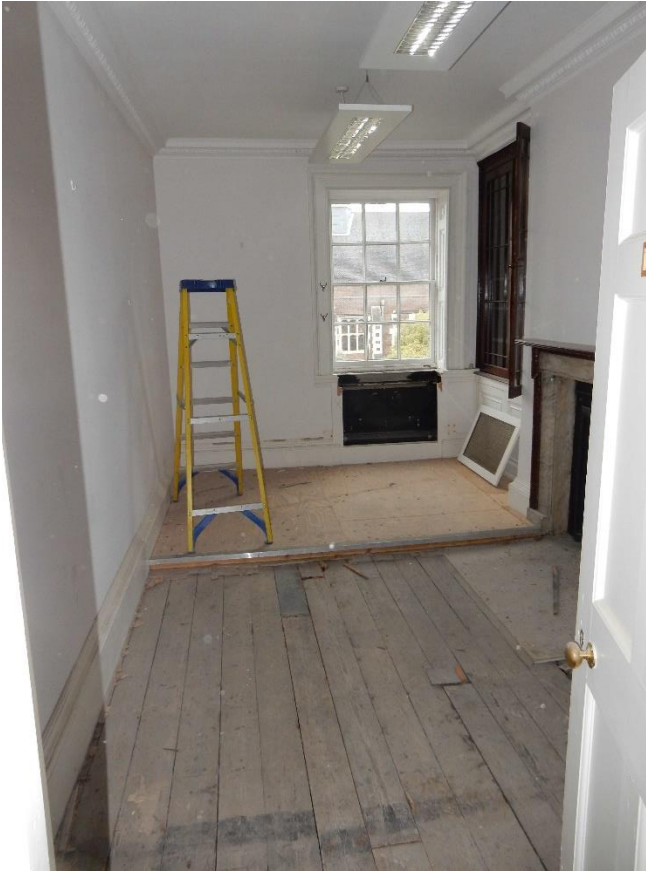
Office 3 – Platform to be removed.
