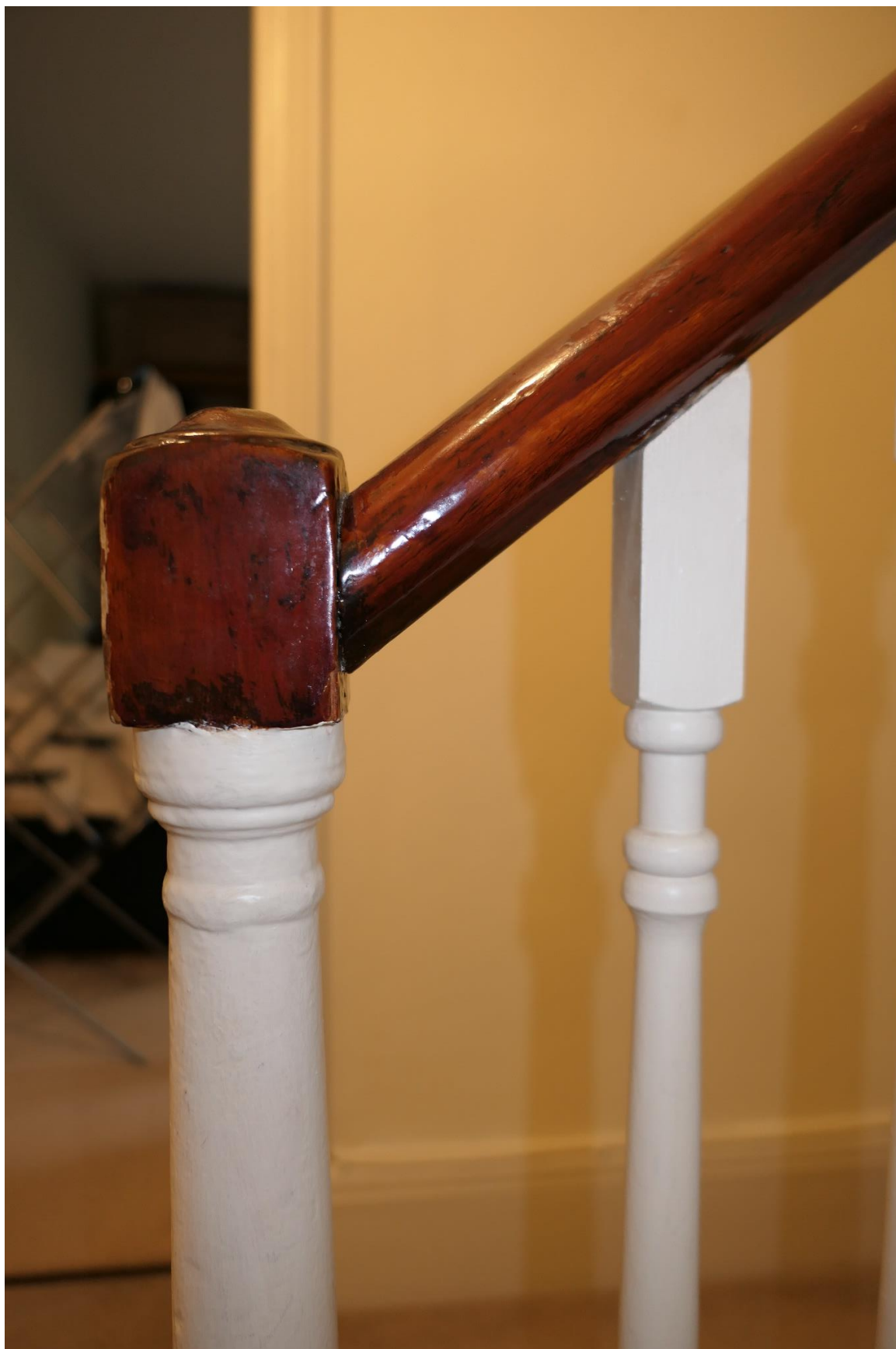
Photo 5: A detail of the original newel post, with the non-original balustrade also seen.
