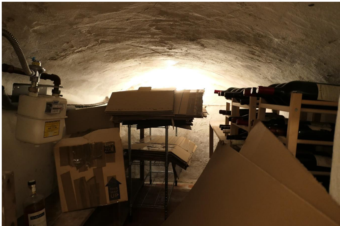
Photo 6: The internalised vault has been tanked with a cementitious render.
