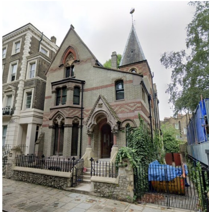
Figure 8: The front façade and flank facades of the building, viewed from Oakley Square.
