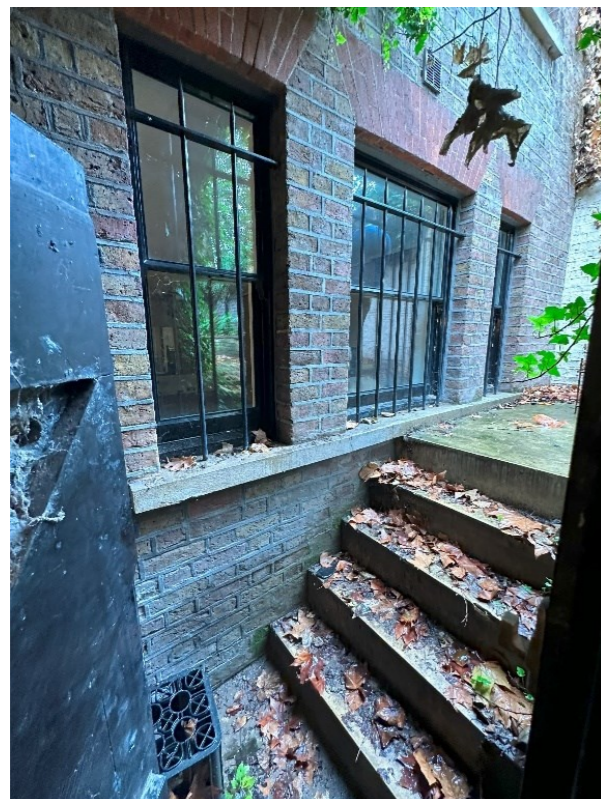
Figures 14: An external view of the steps lower ground floor level.
