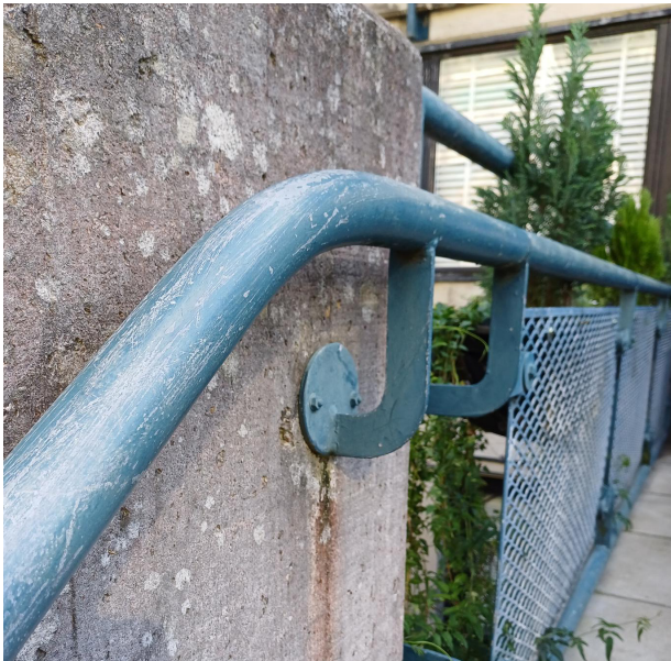
Blue painted metal handrail to external staircase leading to the front of the dwelling with support brackets fixed to concrete wall
