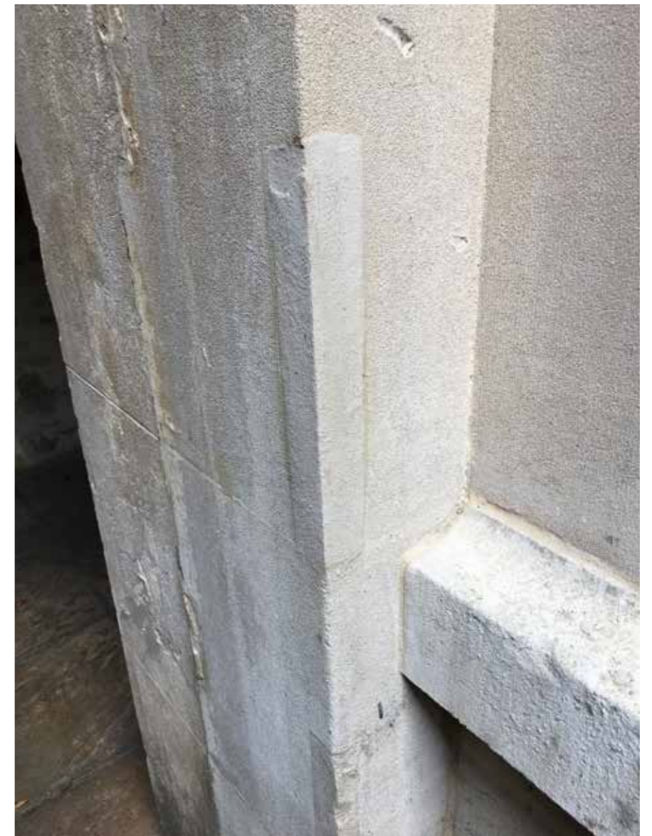
Photo of tinting repair taken on October 23rd, 2024.
