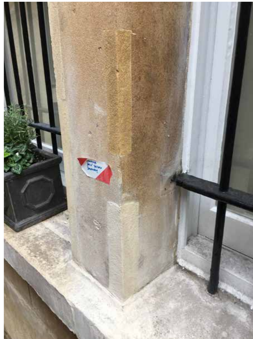
The corner repair after ten days. The repair is considered satisfactory.
