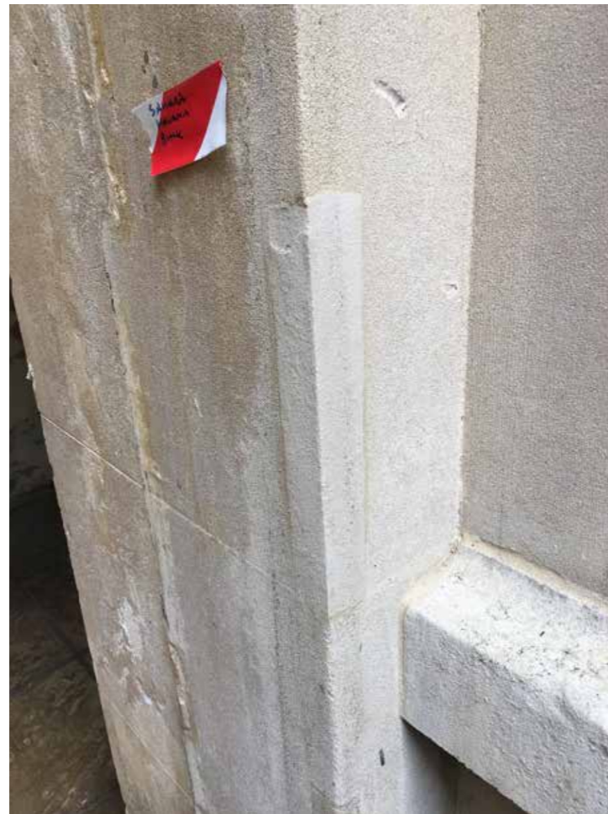
The corner repair after ten days. This repair is considered satisfactory.
