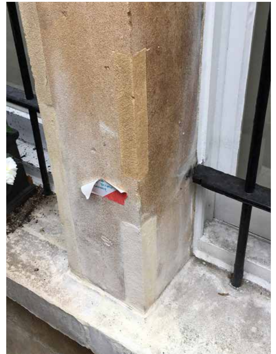
Photo of tinting repair taken on October 23rd, 2024. The repair identification label is still in place.
