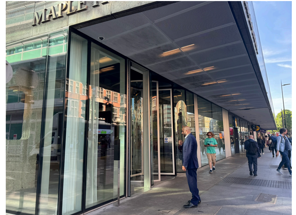
Existing metal mesh soffit with lighting within ceiling void above
