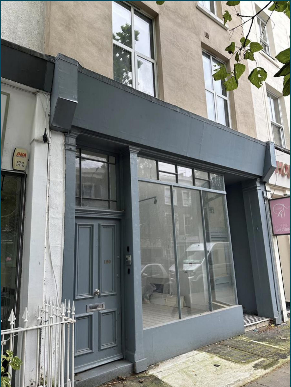
Fig.2 – Photo showing the current external view of the frontage
