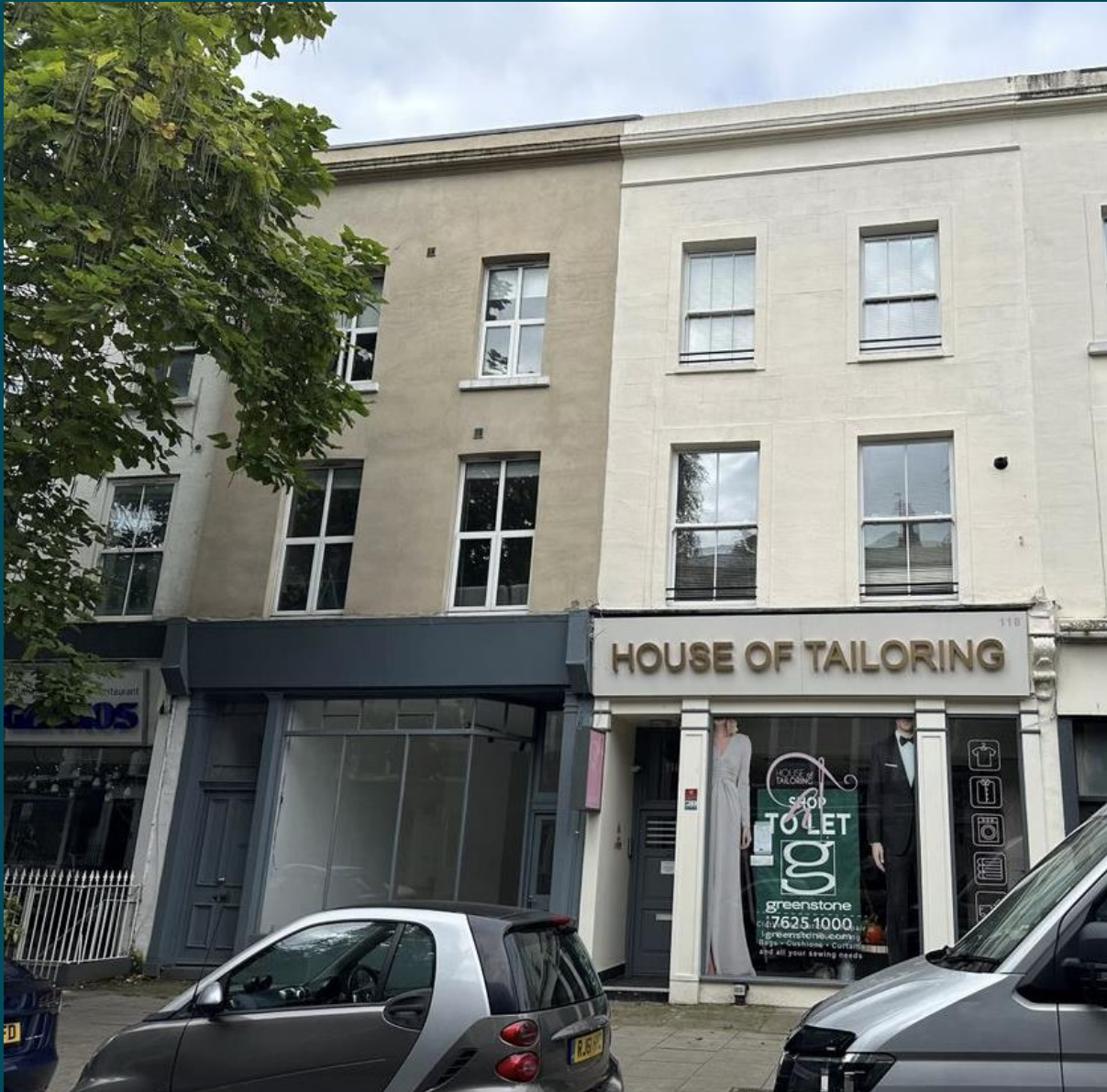
Fig.3 – Photo showing the current external view of the frontage
