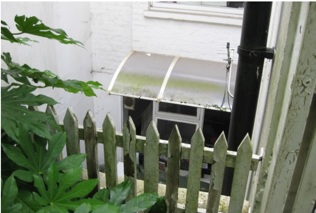
Rear-facing basement level window.
