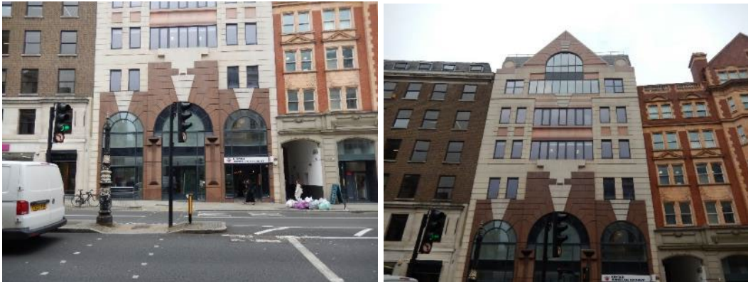
The Site lower level (left, facing) and upper level (right)
