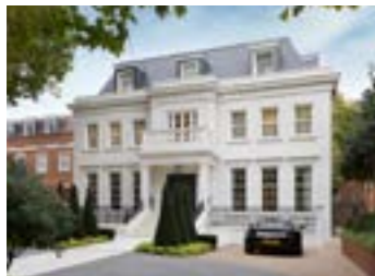
62 Avenue Road Full demolition with basement
