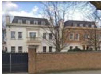
38/40 Avenue Road Full demolition with double basement
