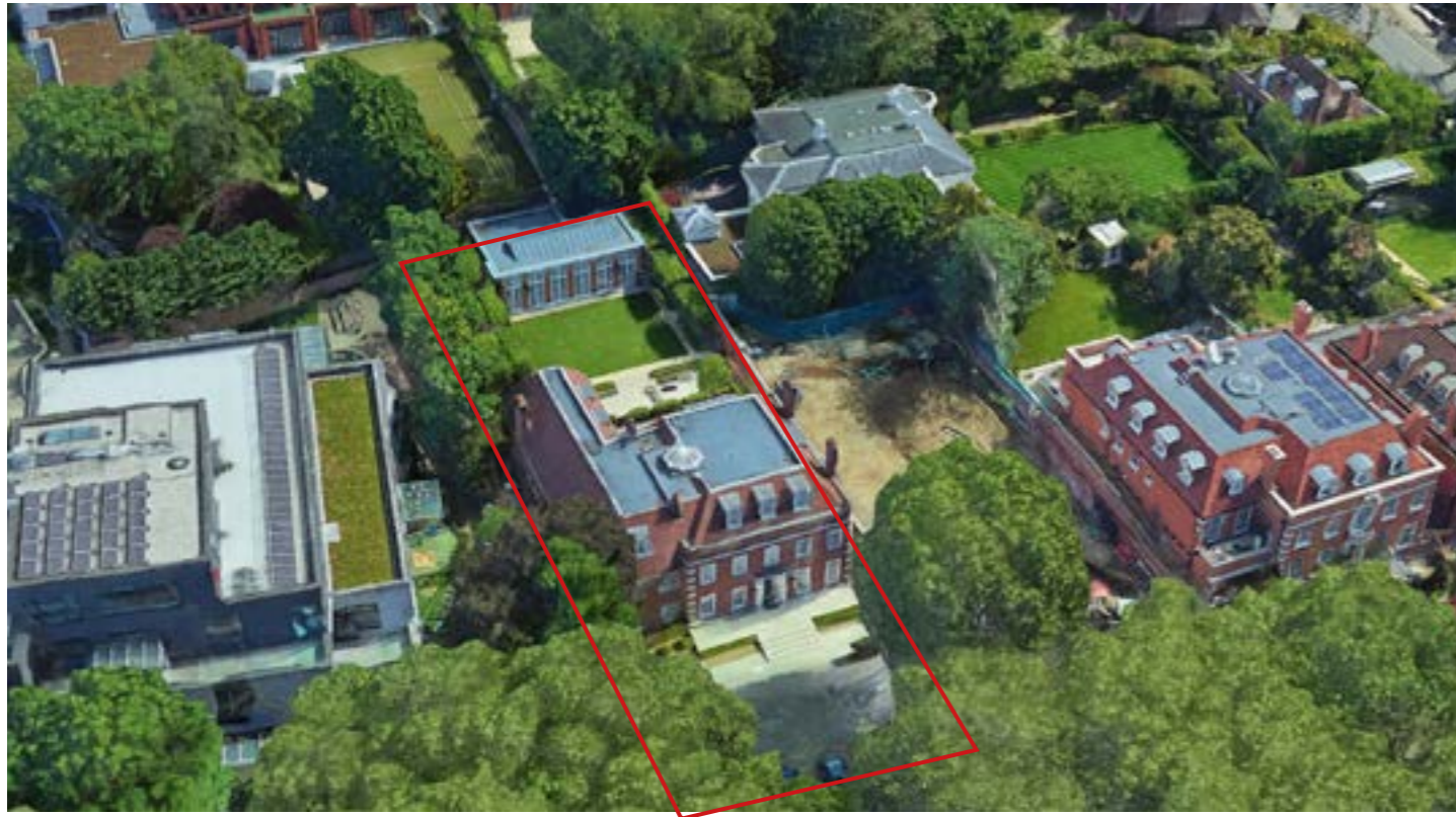
VIEW FROM WEST - FRONT OF PROPERTY
