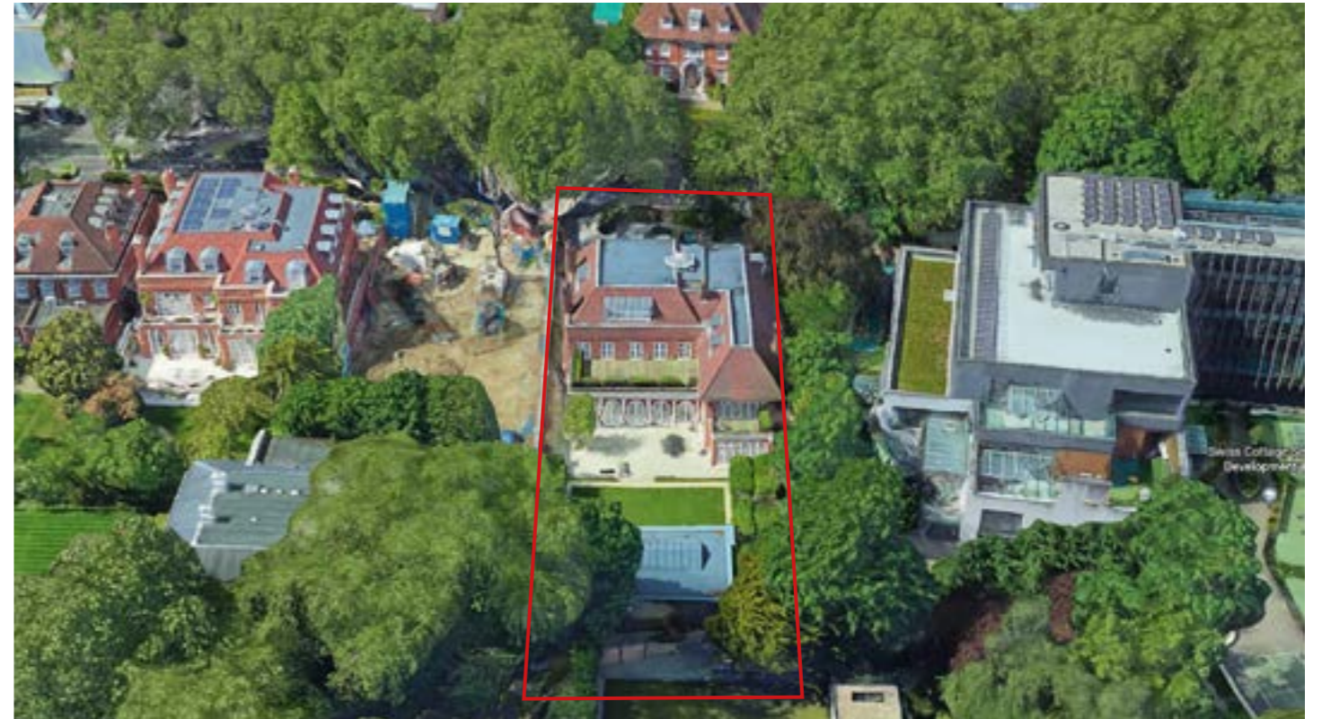
VIEW FROM EAST - REAR OF PROPERTY
